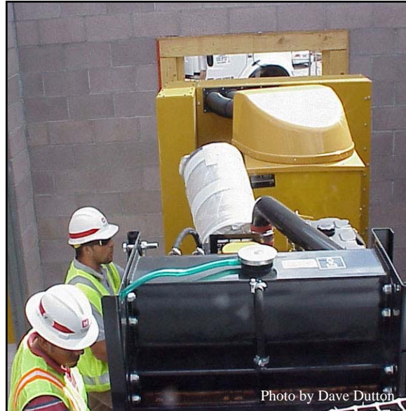
Corps employees install a new generator at Abiquiu Dam that will play the critical role of supplying the dam with emergency power when needed.
