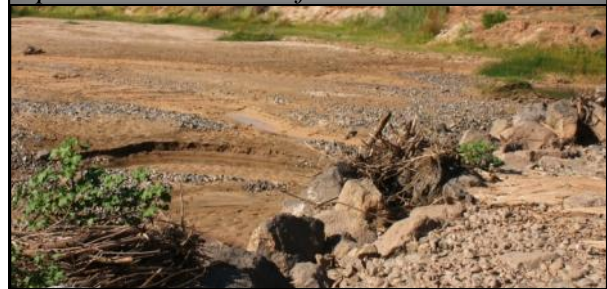
Downstream, the channel has degraded leaving a large drop from the top of the apron to the bottom of the channel.
