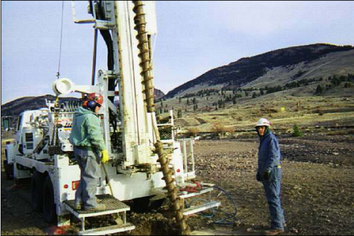
Photograph 5: Removal of Casing at MW19
