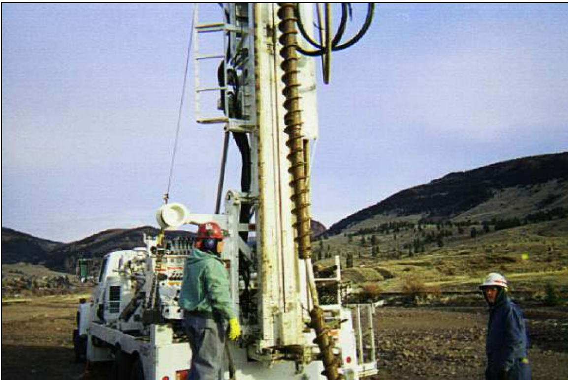
Photograph 6: Removal of Casing at MW19
