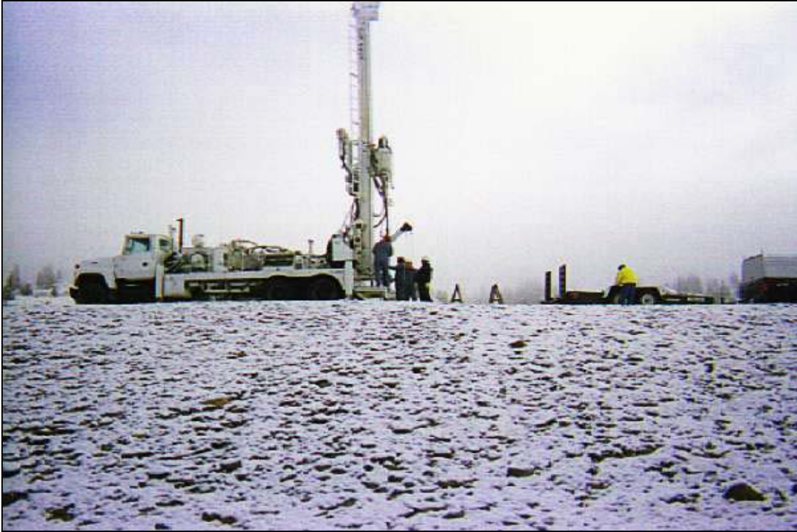
Photograph 15: SB1 from MW11
