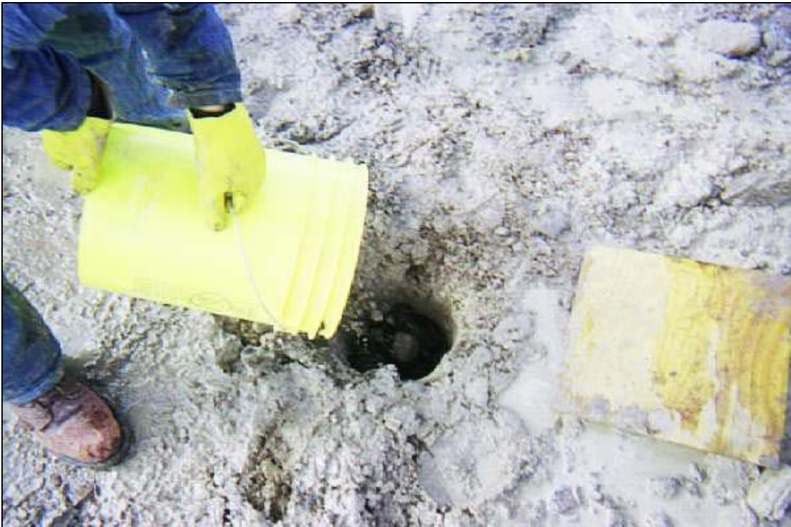
Photograph 18: Placing Bentonite Pellets in SB1
