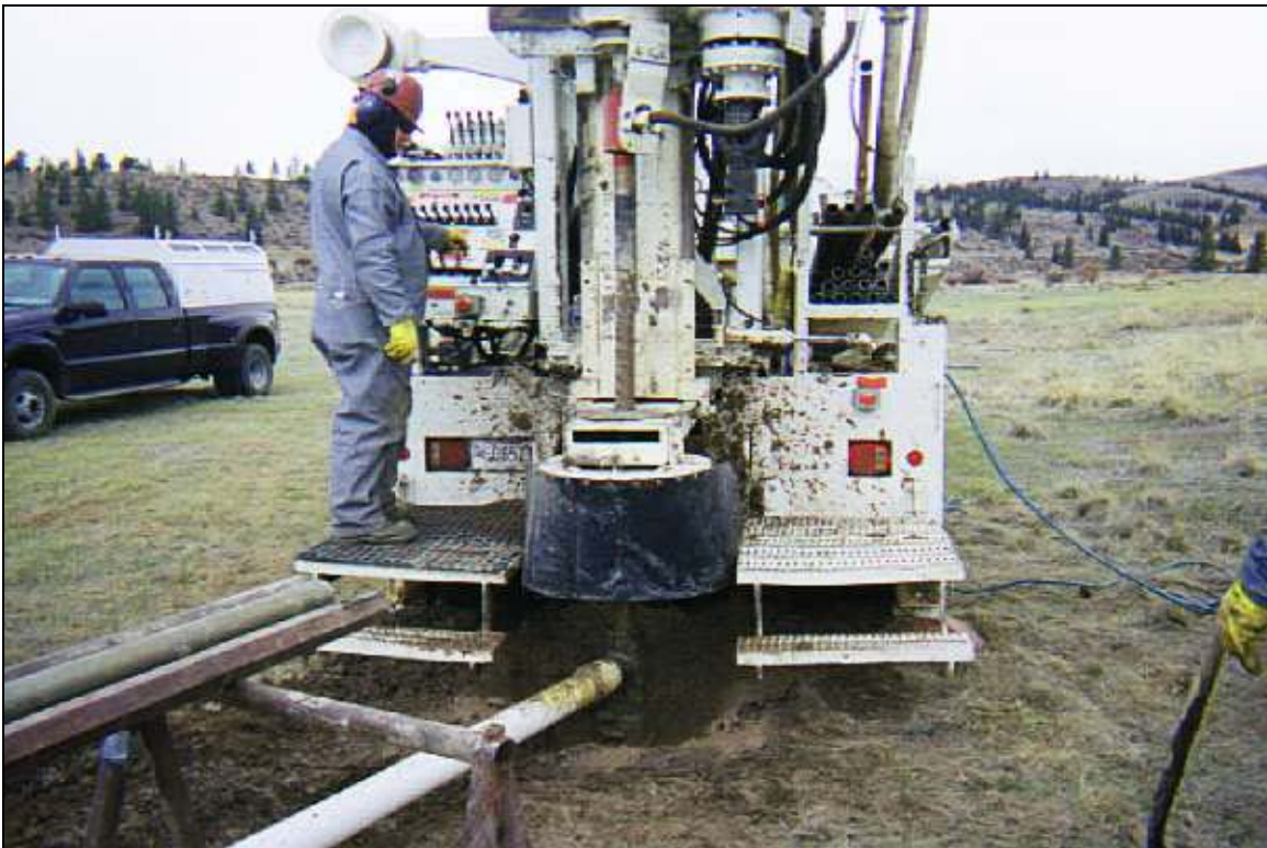
Photograph 12: Blowing out MW18 Boring with Air-Rotary
