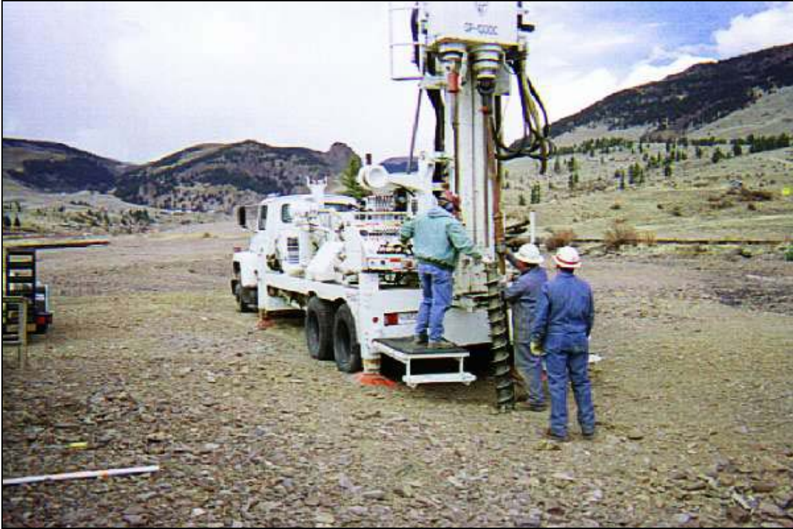
Photograph 3: Setting up at MW19 Original
