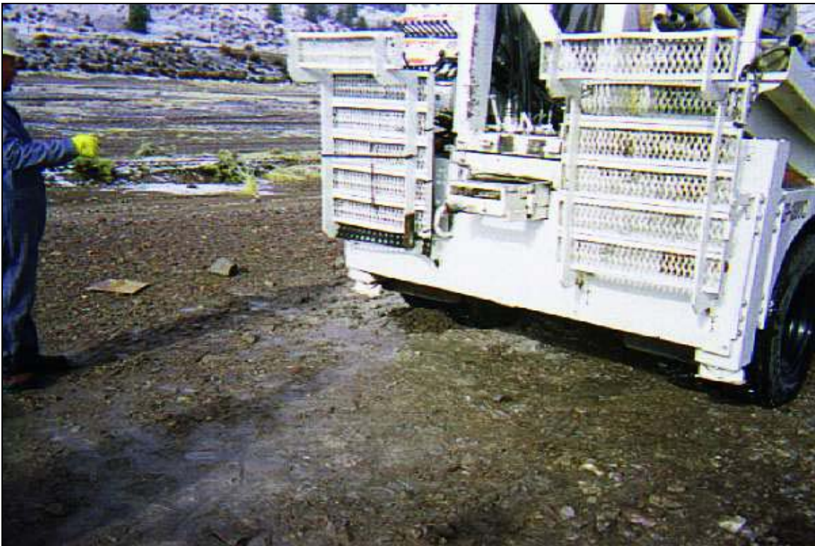
Photograph 20: Cap Material at SB1 Compacted with the Drilling Rig
