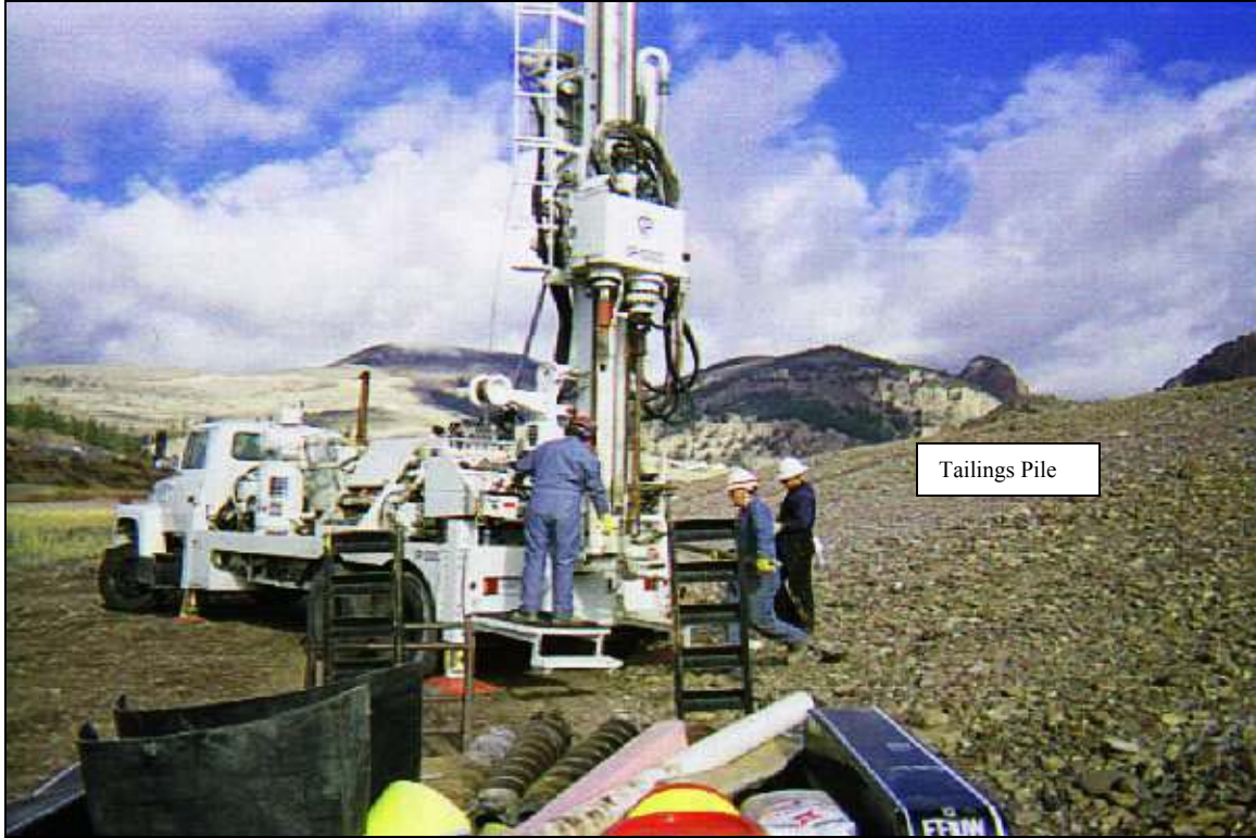
Photograph 21: Setting up at MW16
