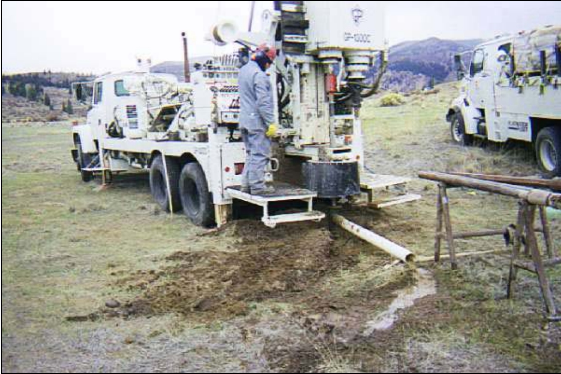
Photograph 11: Blowing out MW18 Boring with Air-Rotary
