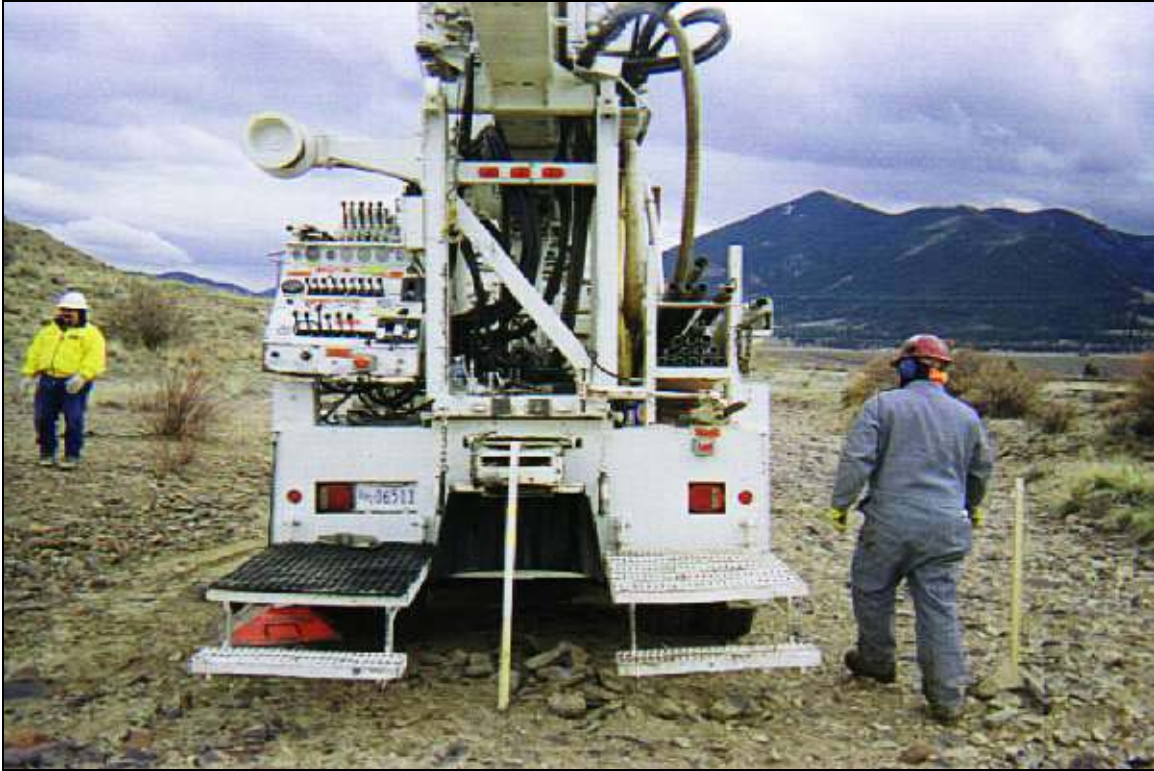
Photograph 13: Setting up at MW17 Location
