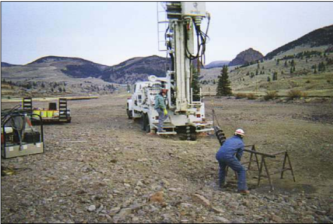
Photograph 4: MW19 Borehole Advancement
