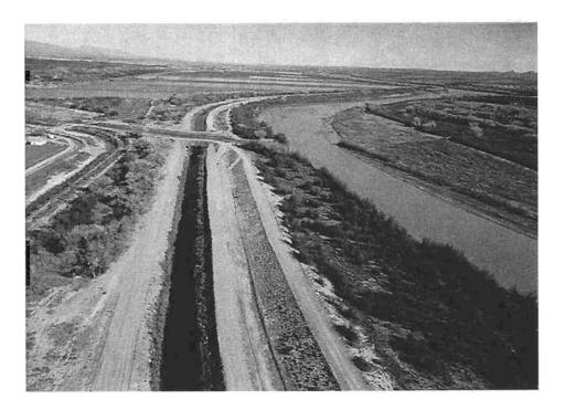
Photo 2 Conveyance Channel and floodway. Note spoil bank levee between the two.
