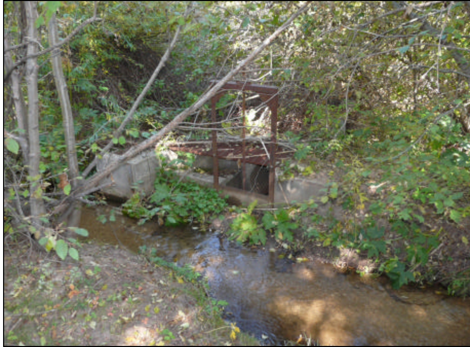
Figure 4.5. Sluice, view to north.
