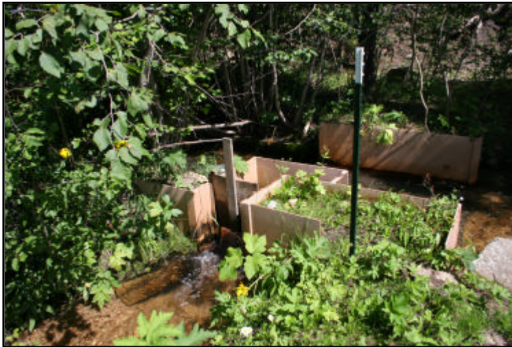
Figure 1-2. Acequia de la Posecion diversion structure – Acequia water diverted toward lower left of photo.
