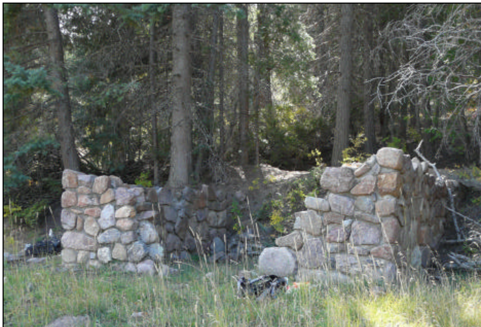
Figure 4.10. Stone structure abandoned during construction.
