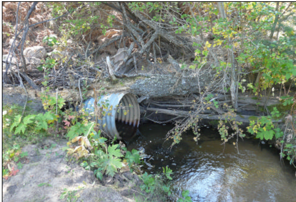
Figure 4.6. Predominant type of culvert, view from upstream.
