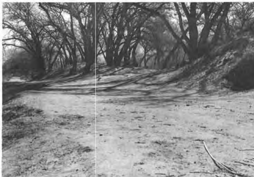
Figure 8. Existing Corrales levee (January 1977)
