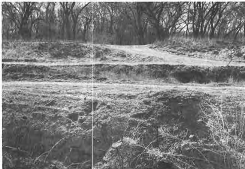
Figure 7. Existing Corrales levee (January 1977)
