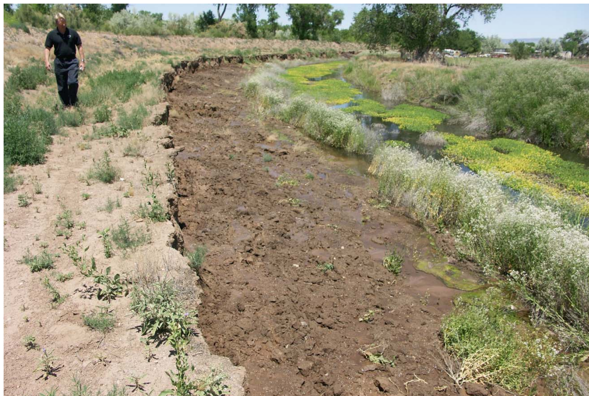
Figure 22 Potential spoil bank failure
