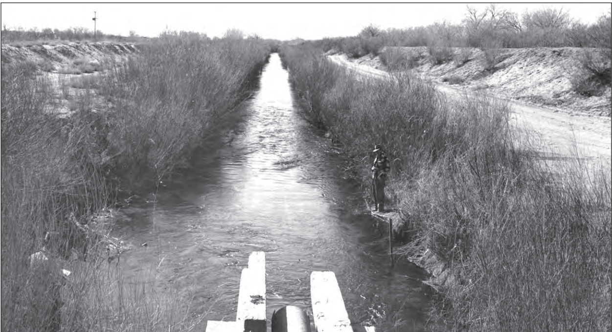
Figure 67. Albuquerque Riverside Drain at the Griegos Heading, 1952. Source: USBR.
