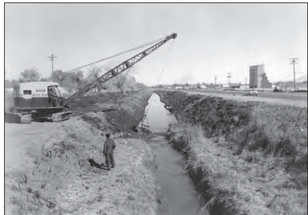
Figure 55. (Bottom Right) Cleaning operations on the Lower Old Jarales Acequia, 1957. Source: USBR.
