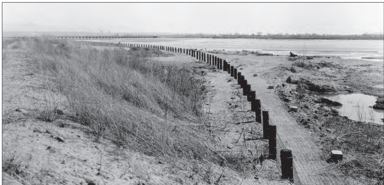
Figure 35. Pilings and wire fencing protecting levee bank near Old Town, 1931. Source: MRGCD.
