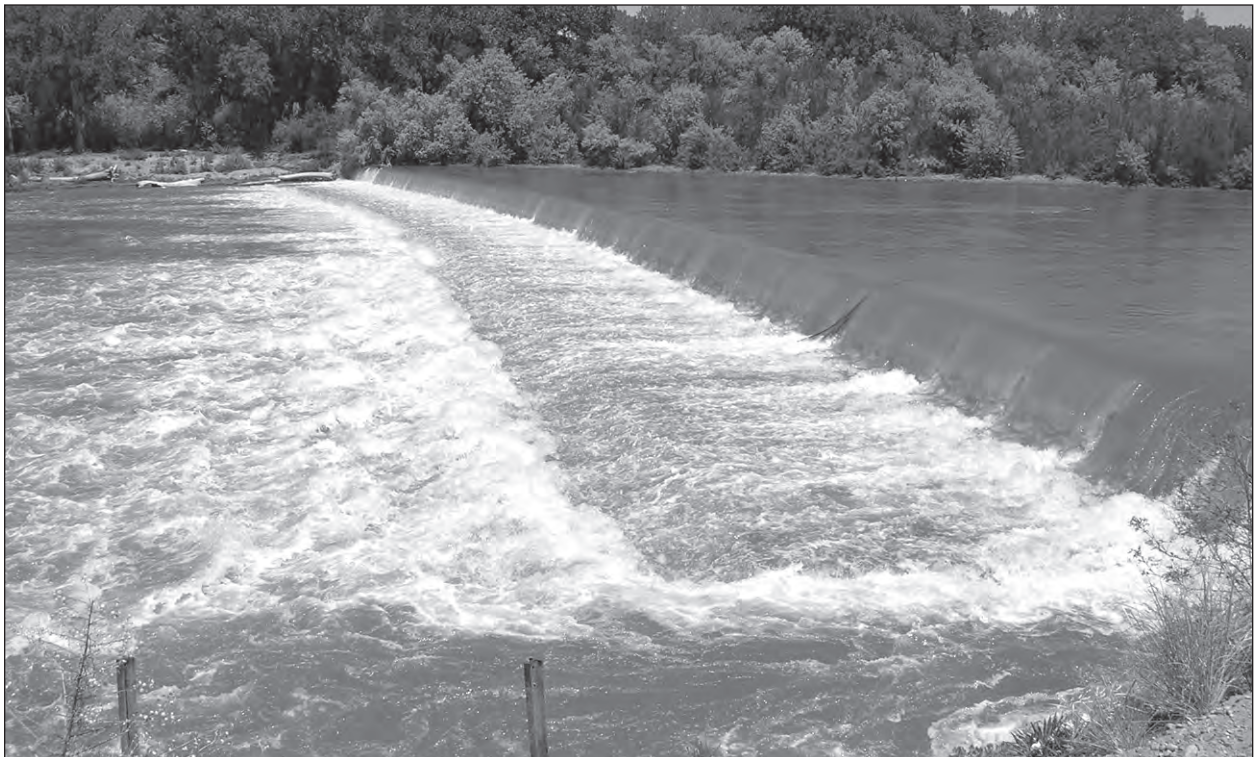
Figure 16. Angostura Diversion Dam, looking west, 2007. Source: VCHP.
