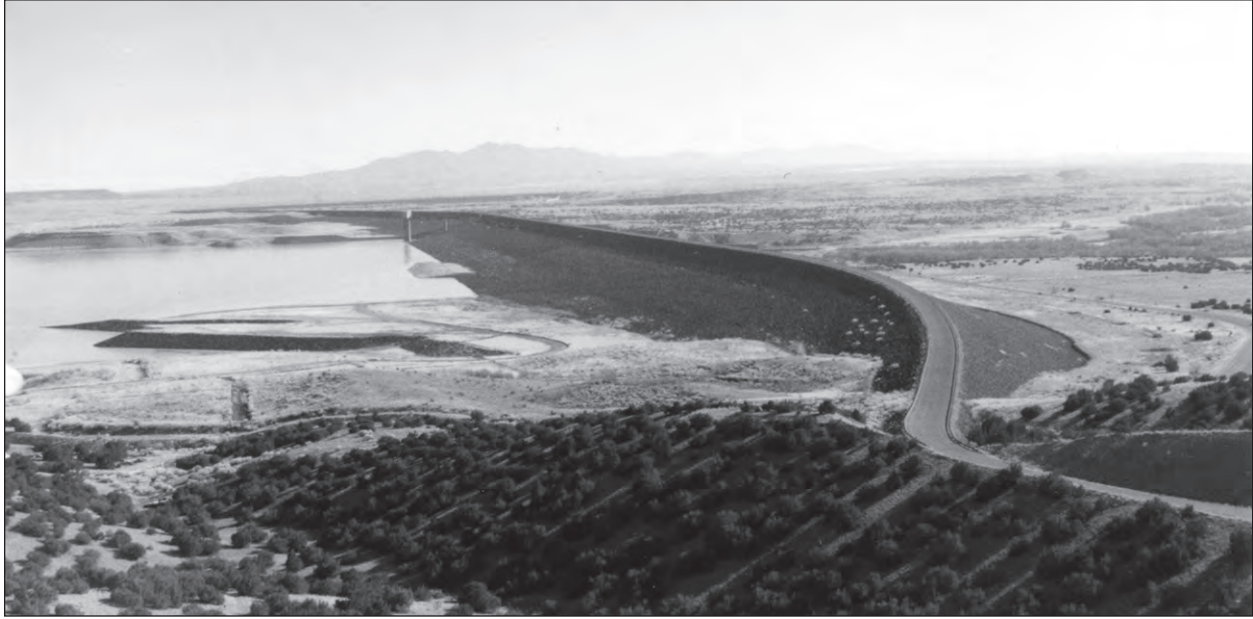
Figure 22. Aerial view of Cochiti Dam soon after completion, looking southeast. Source: USACE.
