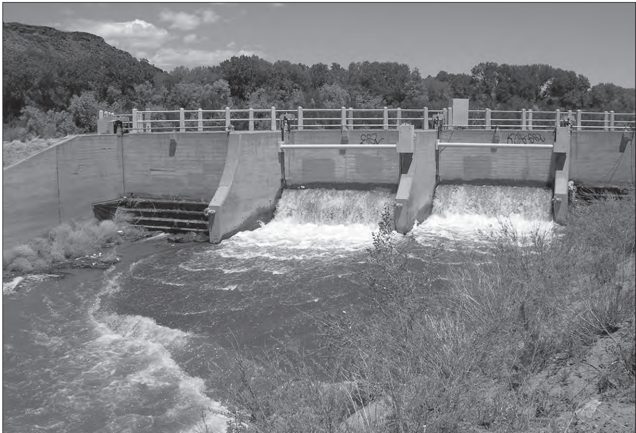
Figure 46. Outlet works at the Angostura Diversion Dam, 2007. Source: VCHP.
