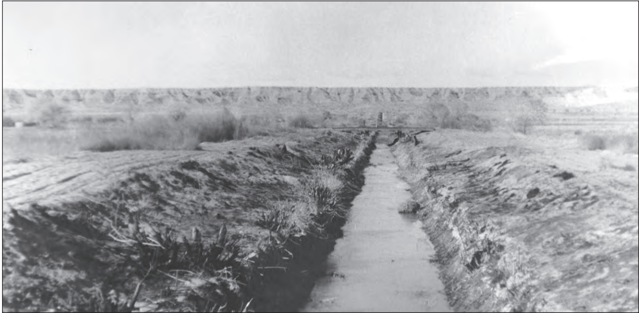
Figure 56. Huning Lateral in the Belen Area showing new concrete check structure, 1957. Source: USBR.
