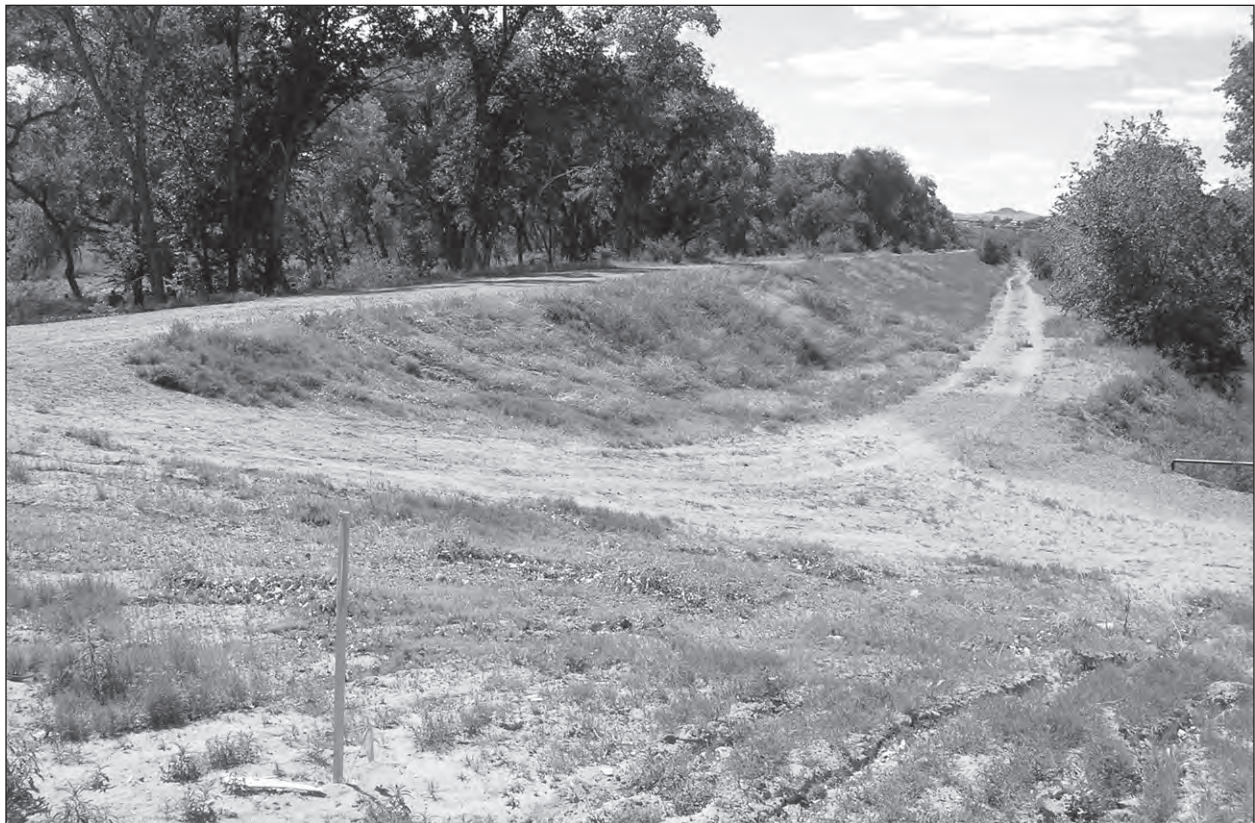
Figure 33. “Engineered” levee just north of Central Ave. Bridge, Albuquerque, 2007. Source: VCHP.
