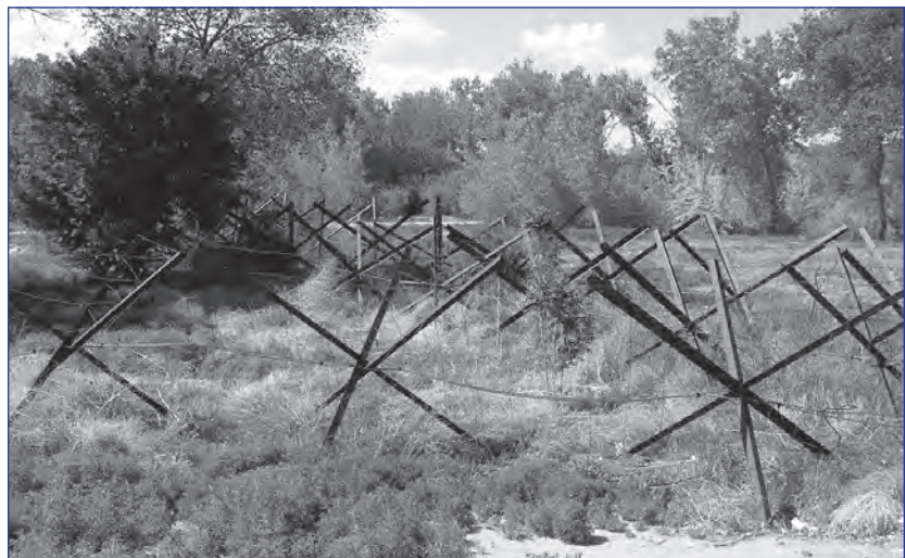
Figure 45. (Right) Kellner jack field north of Central Ave. Bridge, Albuquerque, 2007. The Rio Grande is located behind the line of trees on the right of the photo – some distance from the jetty jack field. Source: VCHP.
