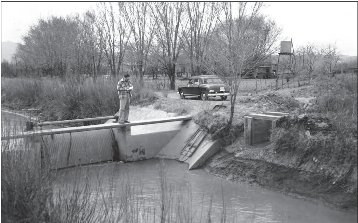
Figure 63. Radial gate check on unidentified lateral in the Socorro Division, 1952. Source: USBR.
