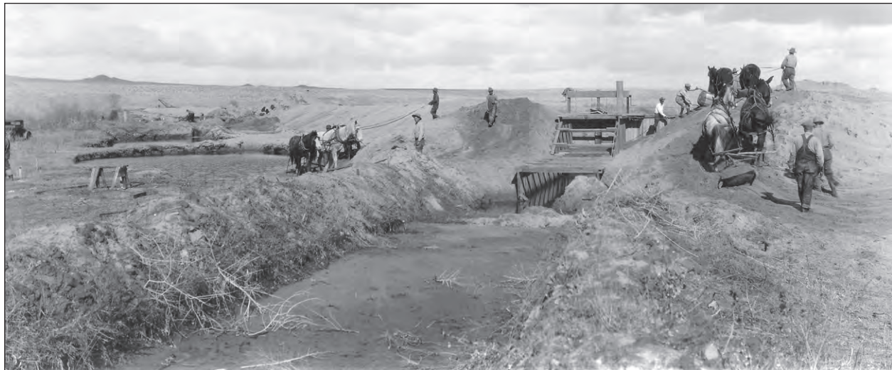
Figure 17. MRGCD irrigation ditch under construction near Laguna cut-off highway (later Route 66), 1931. Note use of horse teams and Fresno scrapers. Source: MRGCD.
