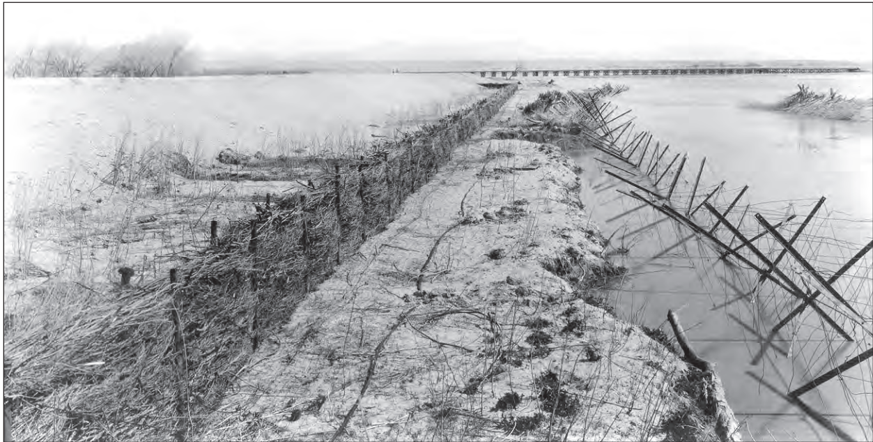
Figure 14. Drawing of levee protection, 1939; Brush protection structure with wire mesh fence on MRGCD levee, 1931. Source: MRGCD.
