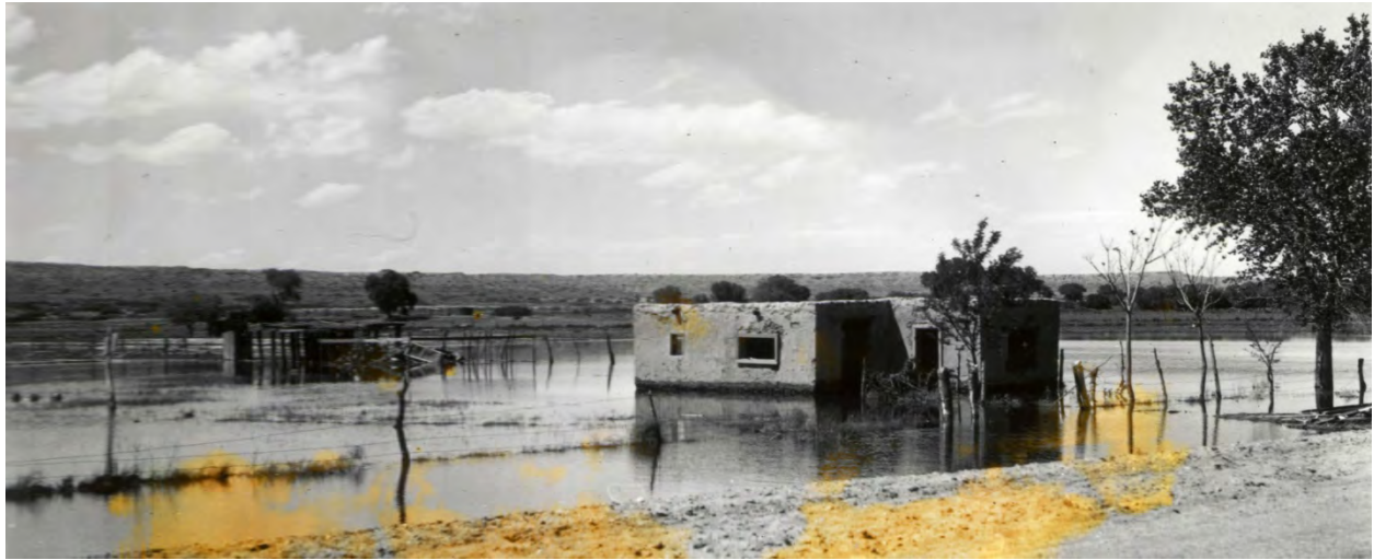
Figure 7 Española Valley floods of 1942 showing ponding and saturation of this structure's adobe walls.
