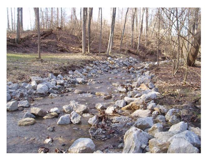
Figure 22 Sorting of trapezoidal riprap channels into rock clasts (Source: Alan Schlindwein).
