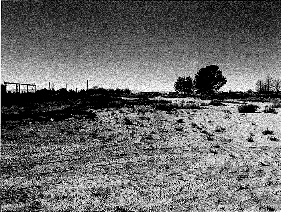
East to west view of proposed storm water pipe route through ROW adjacent to N. Florida Ave.
