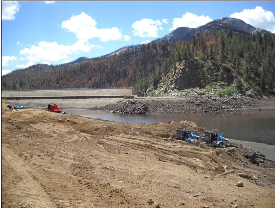
Figure 9. Photograph showing the staging area where fire debris has been cleared and lake side portable pumps have significantly lowered the lake. As lake levels are lowered, the pumps are moved lower. View approximately to S. Photograph No. 4636; 7-30-2012.
