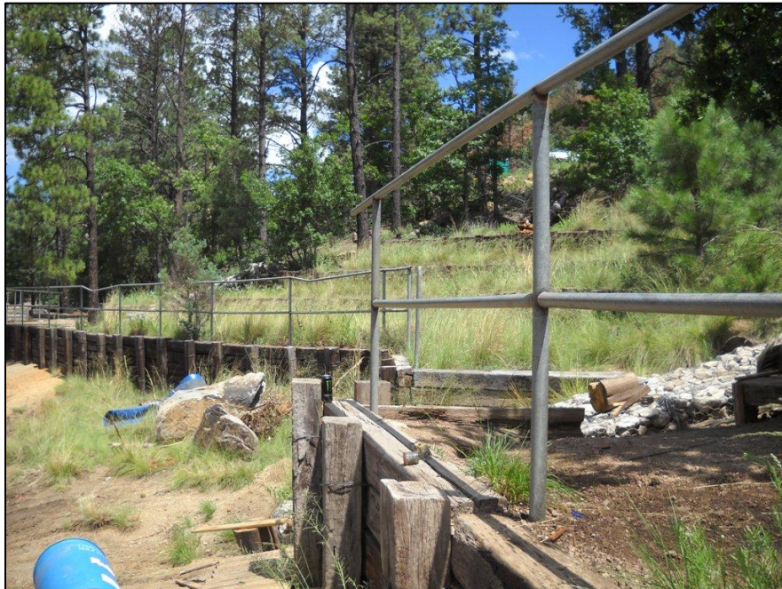
Figure 7. Photograph showing railroad-ties for hill slope stabilization, rock-filled gabion baskets for roadside rainwater drainage, and hand-railing for public access to the Bonito Lake shoreline. View approximately to N. Photograph No. 4631; 7-30-2012.
