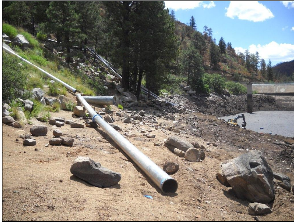
Figure 10. Photograph showing the piping from the pumps that carry water to the Bonito Lake road surface to be delivered downstream. Backhoe in the background is installing a pump closer to the lakeshore. View approximately to SE. Photograph No. 4621; 7-30-2012.
