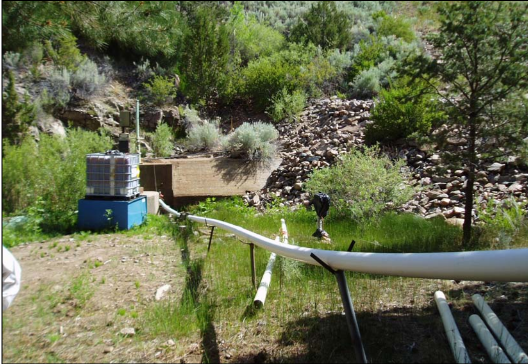
Figure 4.1 Diversion structure showing toe of Nichols Reservoir, intake water control structure to be left in place, and pipeline running uphill to existing ditch.
