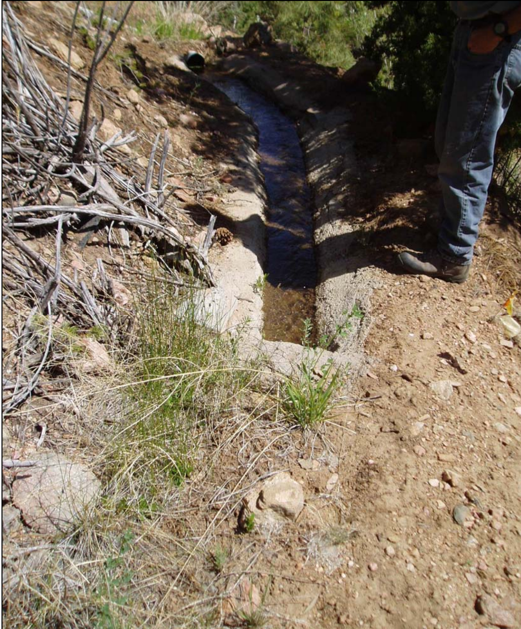
Figure 4.5 View of partially buried, partially concrete-lined portion of the acequia.
