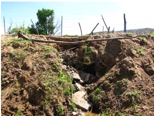
Severe erosion on existing non-reinforced acequia, May 2009.
