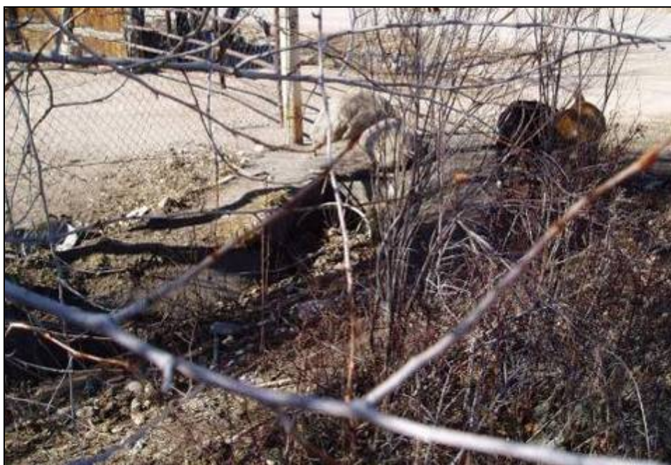
Figure 4.29. Culvert / siphon carrying ditch under road.
