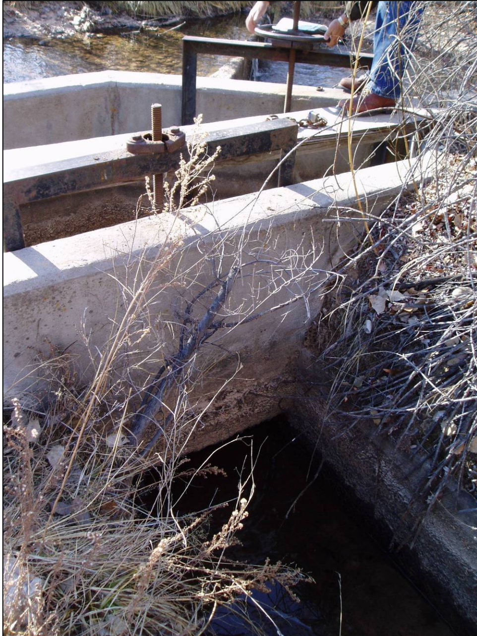
Figure 4.10. View of the second sliding metal gate shown in Figure 4.9, from opposite direction (facing south), showing water flowing into concrete-lined ditch (foreground). Note removable wheel attached to headgate mechanism in background.
