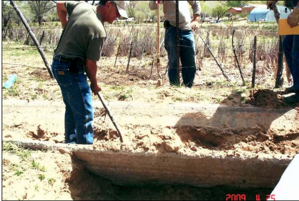
Figure 4.42. Ditch cleaning operations due to ditch overflow (note erosion in foreground). Photograph courtesy of Beraldo Montoya.
