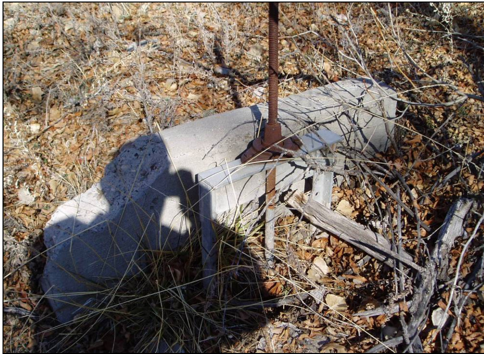
Figure 4.14. View of former Quemado headgate, facing northwest, showing gate mechanism.
