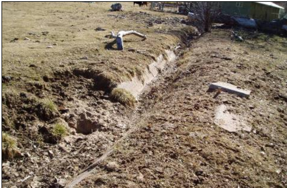
Figure 4.39. View of portion of acequia with extensive trampling and erosion due to cattle. Note displaced fragments of concrete ditch lining to the right of the ditch.
