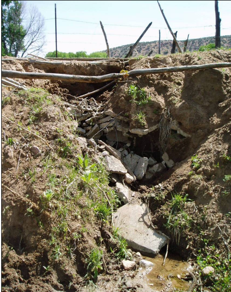
Enclosure 7. Severe erosion undercutting concrete lining, causing it to fail. Erosion also severely impacts the raised berm on which this part of the ditch runs.
