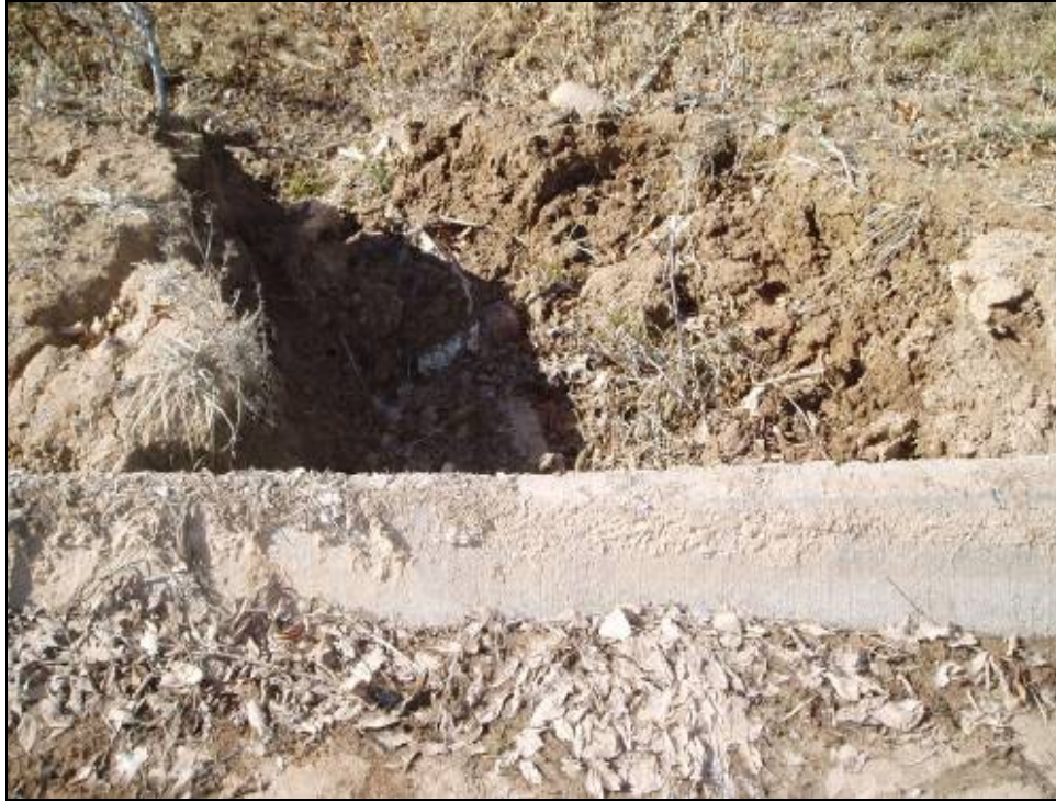
Figure 4.38. Example of erosion undercutting concrete lining due to trampling by livestock.
