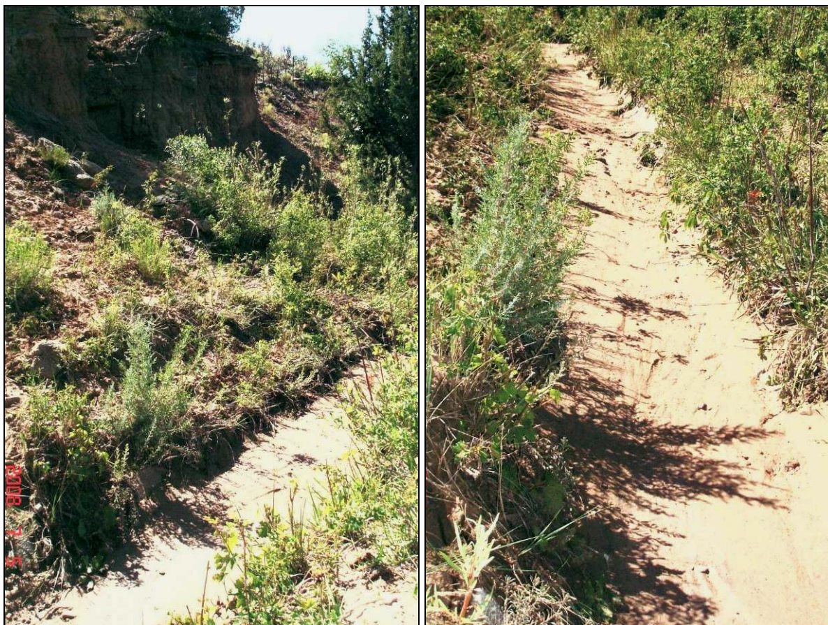
Figure 4.36. Views of acequia completely full of sediment washed in from adjacent slope. Photographs courtesy of Beraldo Montoya.
