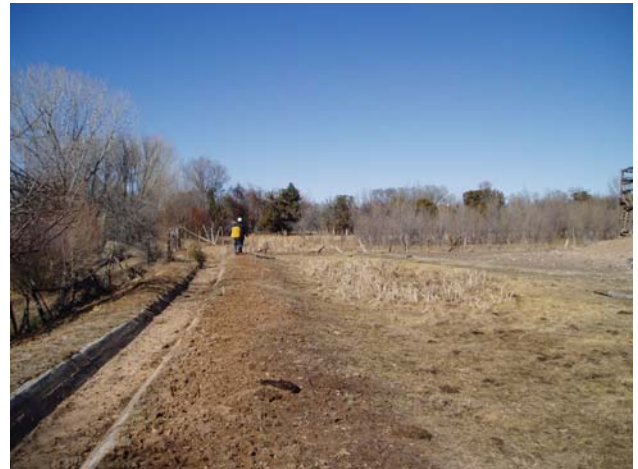
Existing non-reinforced concrete acequia, January 2009.
