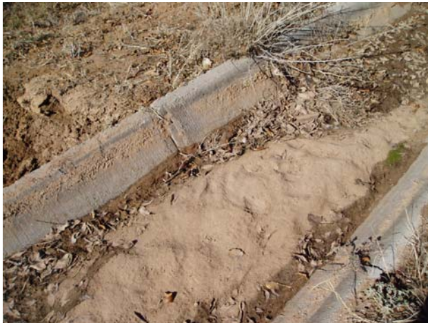
Existing non- reinforced concrete acequia showing sediment deposition, January 2009.
