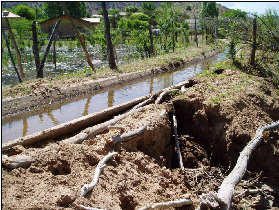
Figure 4.41. Another view of erosion caused by ditch blockage, facing east.
