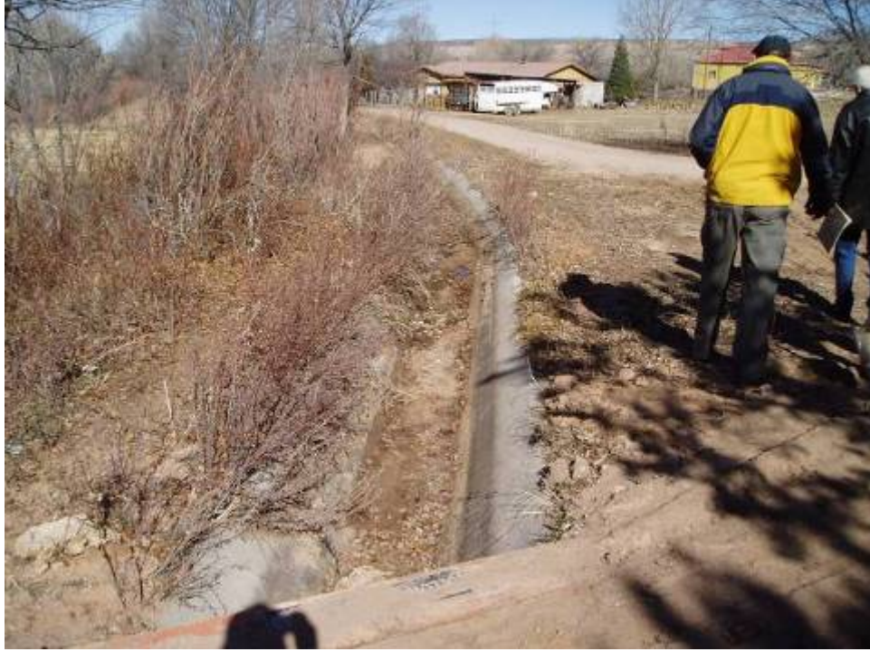
Figure 4.21. Segment of ditch with concrete lining dating to 1986, facing northwest.
