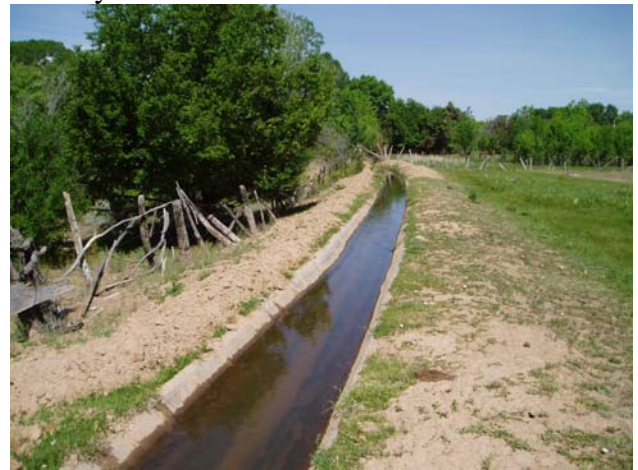
Existing non-reinforced concrete acequia after annual cleaning, May 2009.
