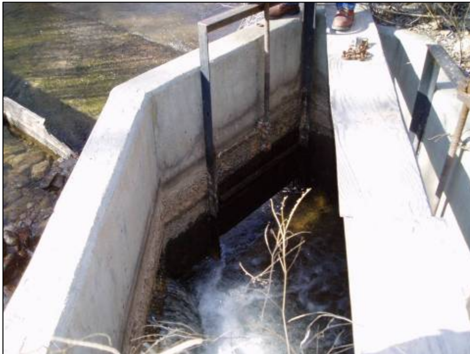
Figure 4.8. View of the headgate of the Acequia de los Ranchos, facing southwest. Note headgate leading into open chamber / sluice box, with second gate leading to ditch (right). Note water pouring in through an irregular opening in the wing wall just to the left of the formal sliding gate.
