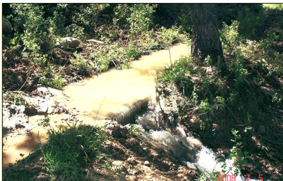
Figure 4.37. Water overflowing ditch as a result of infill of sediment from upslope erosion. Photograph courtesy of Beraldo Montoya.
