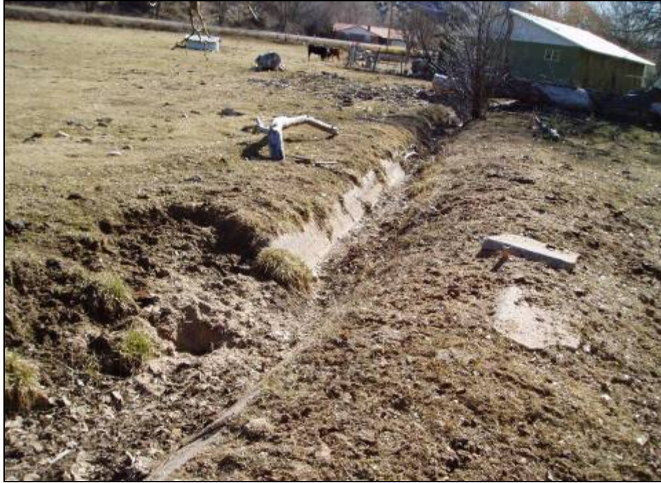
Enclosure 6. View of portion of acequia with extensive trampling and erosion due to cattle. Note displaced fragments of concrete ditch lining to the right of the ditch.
