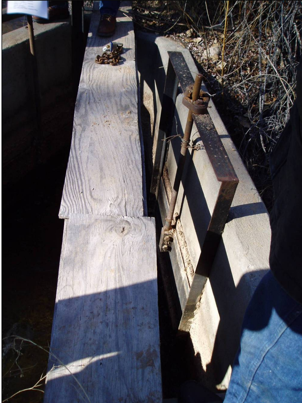
Figure 4.9. Metal gate leading from concrete chamber to ditch channel, facing southwest.
