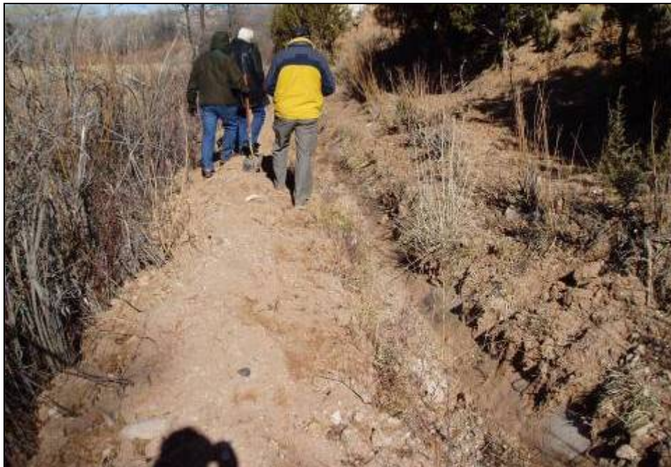
Enclosure 5. View of acequia channel where impacted by downslope erosion, facing northwest.
