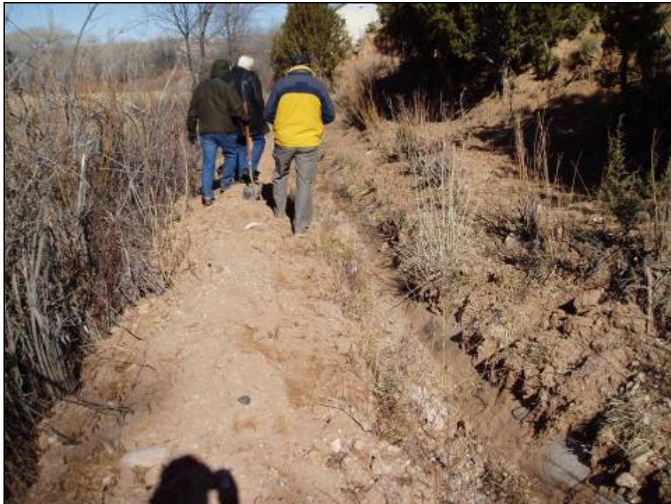
Figure 4.35. View of acequia channel where impacted by downslope erosion.
