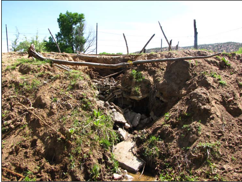
Figure 4.40. Berm erosion caused by ditch blockage and overflow, facing northeast.
