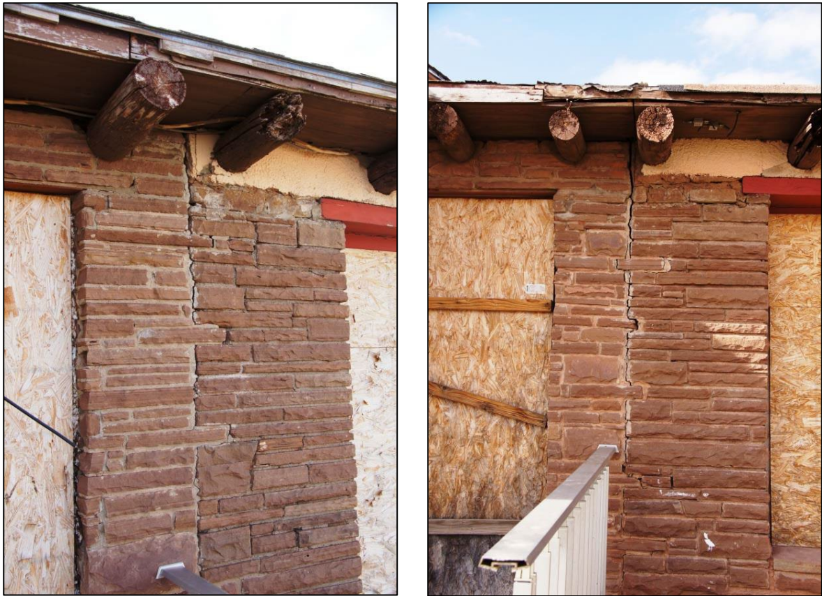
Figure 6. Original sandstone walls to the left, and right side of the juncture crack. Note the heavier mortar joints and lesser craftsmanship of the veneered addition. (Photo: K. Hill, May 2012)
