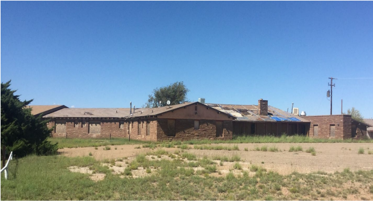
Existing Conchas Lodge Site Condition:
