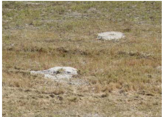
Figure 2.41 Evidence of sandboils. (IN)
