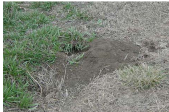
Figure 2.20 Animal burrow in a levee. (IA)
