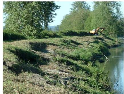
Figure 2.3 Slope failure on bank protection project. (WA)
