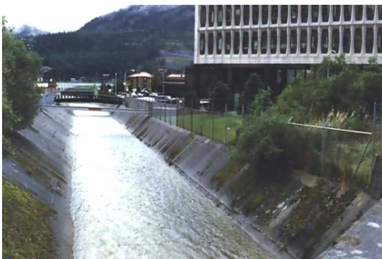
Figure 2.74 ACCEPTABLE concrete lined channel. (AK)
