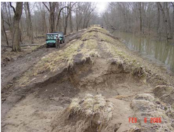
Figure 6.2 and 6.3, Levee breaches along the Wabash River
