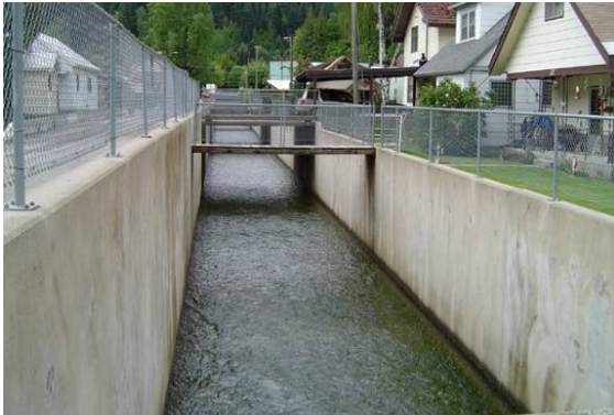
Figure 2.72 ACCEPTABLE concrete lined flood control channel. (ID)
