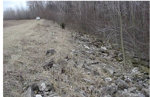
Figure 2.28 UNACCEPTABLE . Tree and sapling growth is well established within the riprap protection on an earthen levee. This overgrowth must be removed. (MO)
