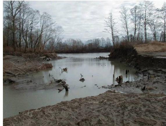
Figure 6.1, Levee breach in Lynden, WA
