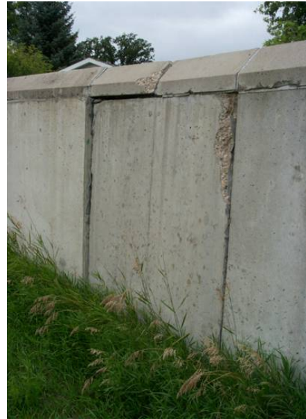
Figure 2.49 UNACCEPTABLE monolith movement in floodwall. The monolith shown in the photo has tilted about 6 inches riverward as well as vertically. Note the movement when compared to the adjoining monolith and the top cap. As the monolith moved considerable spalling has occurred along the joint. This project is monitored very closely during flood events. (ND)
