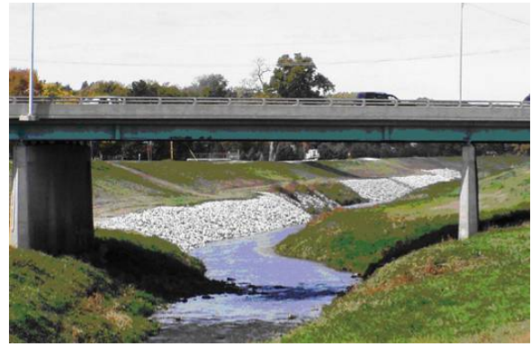
Figure 2.26 ACCEPTABLE riprap for erosion control. (NE)
