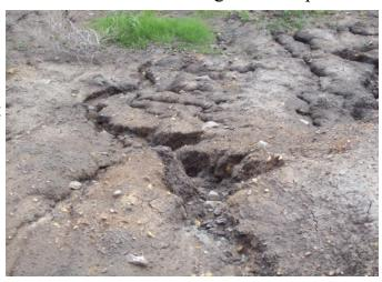
**CHANGE IN SLOPE:** When steeper grades change into shallower grades, they can be subject to vulnerability during times of flood. The change in slope causes a change in velocity and can cause erosion of the soil.
