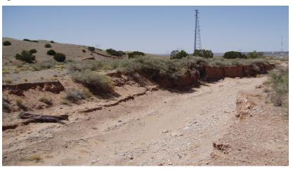
**Scour:** Occurs when the current velocity against the levee is adequate to remove levee embankment materials. Scouring will most likely develop at road crossing ramps and locations where pipes, sewers, and or other structures penetrate the levee.
