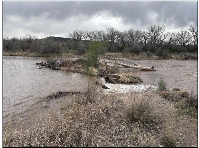
Figure 2. Acequia Salazar diversion dam on Rio Chama
