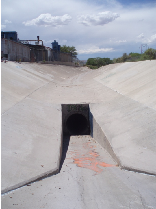
P1: Looking west (downstream) at low flow diversion intake location
