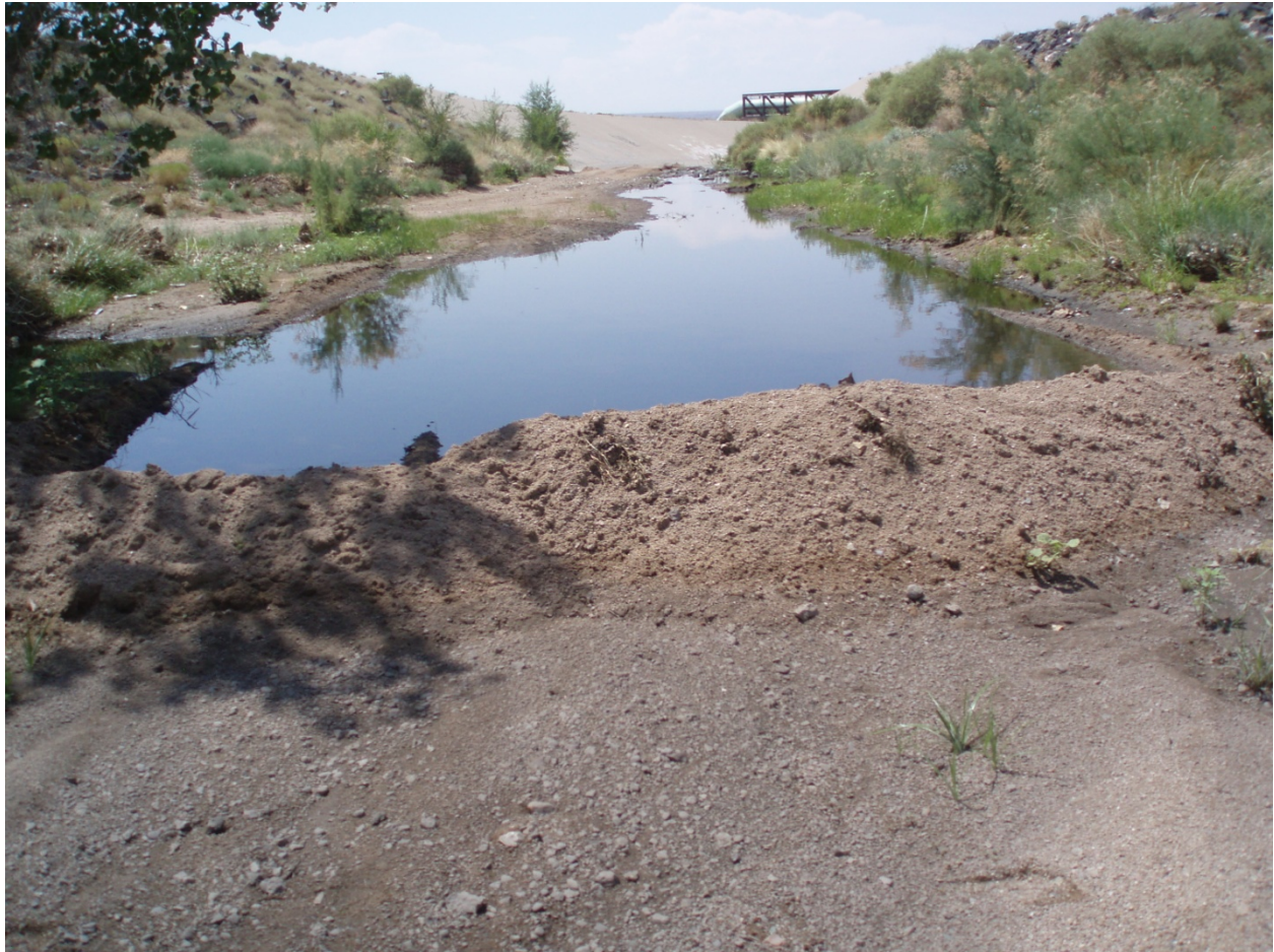
P13: Looking west (downstream) at Pino/NDC confluence. Note earthen berm placed in flow path. Water on D/S side of berm is the result of the berm being flanked by flow. Flow continues into the NDC. This water was discolored as that in P6.
