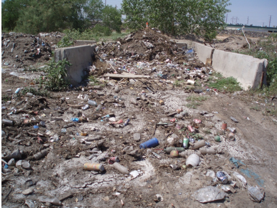
P7: Looking west at debris bins. Note loose, unconfined trash, cracked soils from prior ponding
