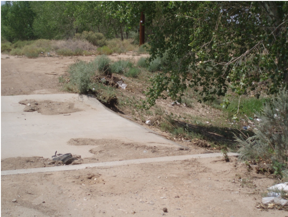
P2: Looking west across trash removal pond's concrete emergency spillway
