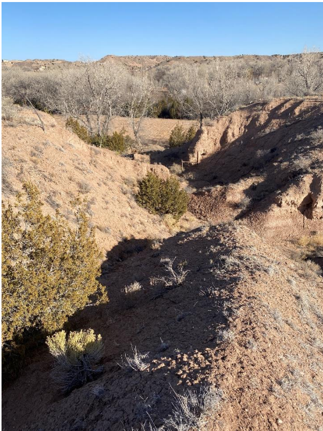
2. Top Left of the arroyo looking North downstream towards the embankment.
