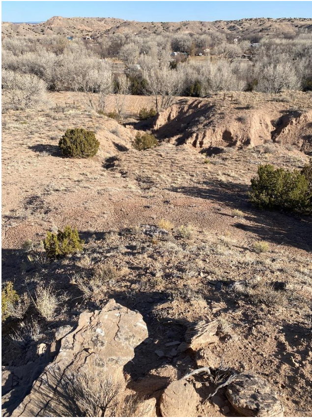
1. Top of arroyo looking north downstream towards the embankment.
