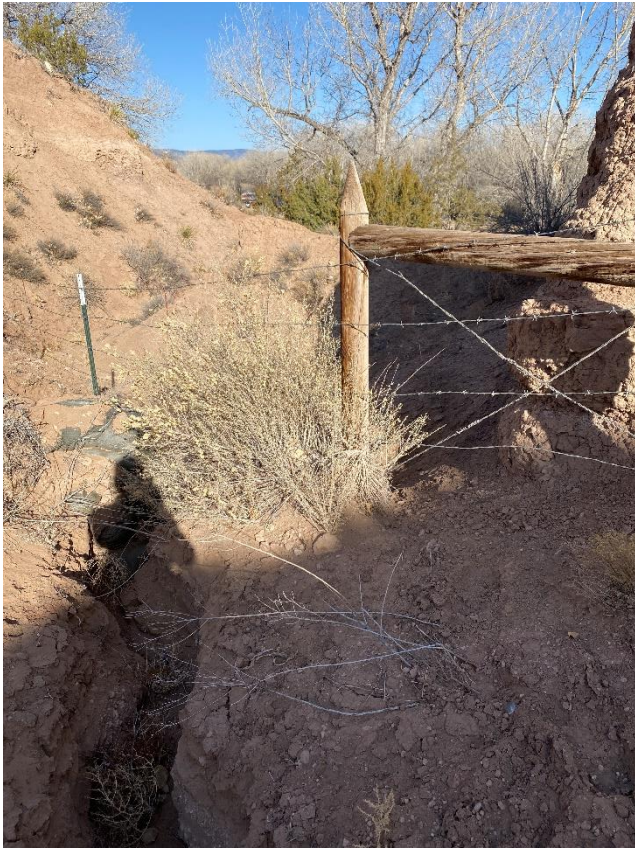
3. Looking South, upstream from the bottom of the arroyo.
