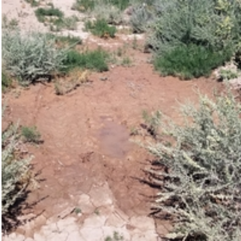
Photo 3: S-01 top of bank, facing east
