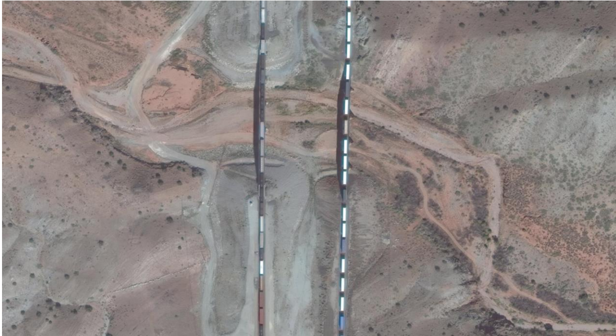
(Figure 4) BNSF Railway ~1,500 linear foot project study area; Digital Globe satellite imagery; September 29, 2019.
