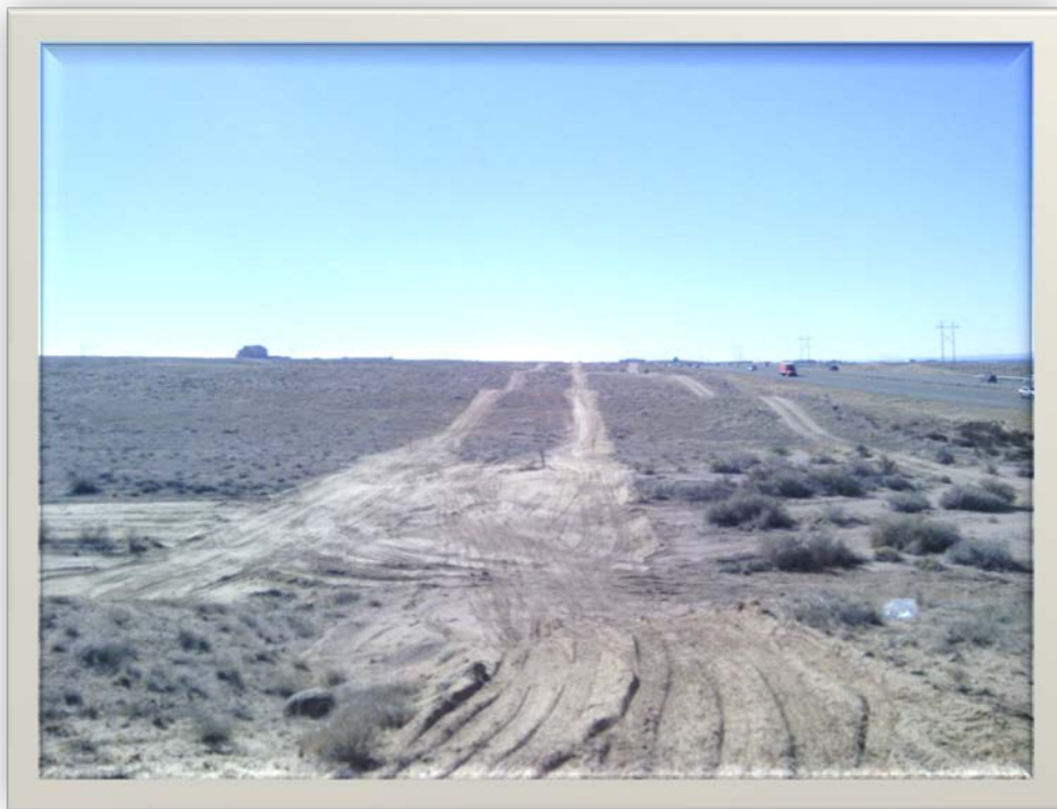
Photo 16: Looking at disturbed corridors crossing arroyos on the east side of I-25
