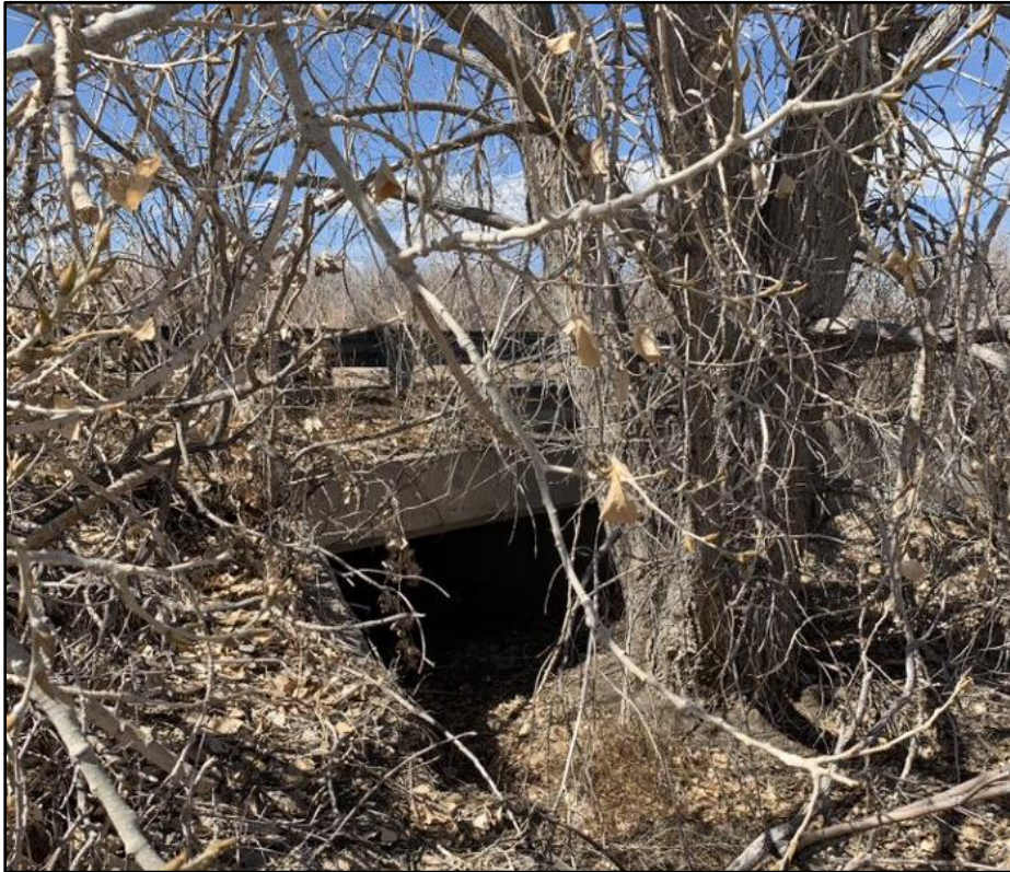
Photograph C-3: View from east side of bridge, facing northwest.
