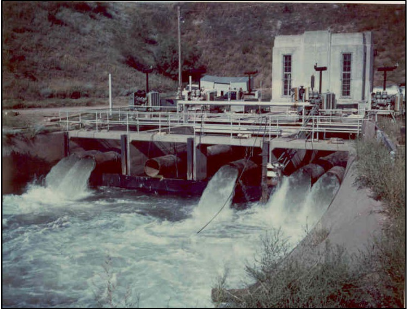
Photo 6-1 Conchas Dam Irrigation Outlet Works
