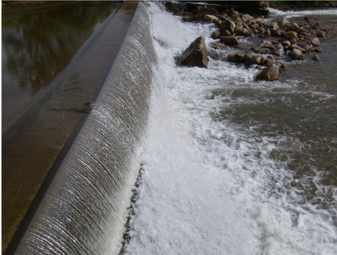
View of weir looking north along downstream side of weir.
