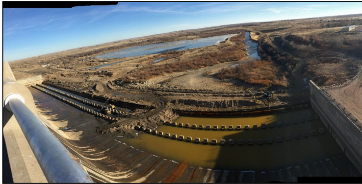
John Martin Dam, Colorado, Stilling Basin Dewatered
