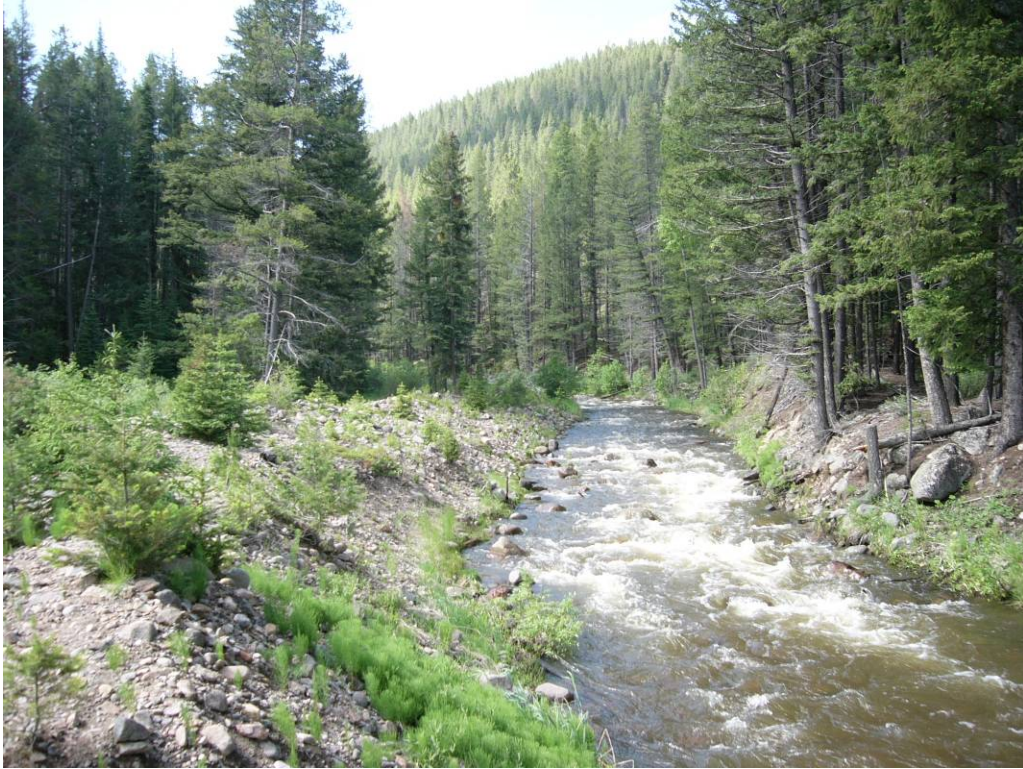
From right bank near opposite of XS#6 looking upstream at rock berm, looks to be built of river sediment with gravel and cobbles.
