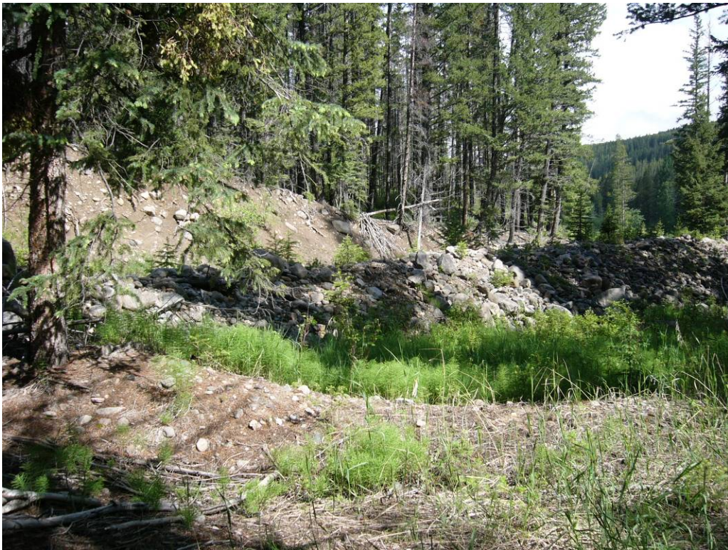
On right bank near upstream end of possible diversion to wetland, toe of left bank hill slope starts just upstream, dike height decreases to about 4 ft in this area (8 ft d/s).
