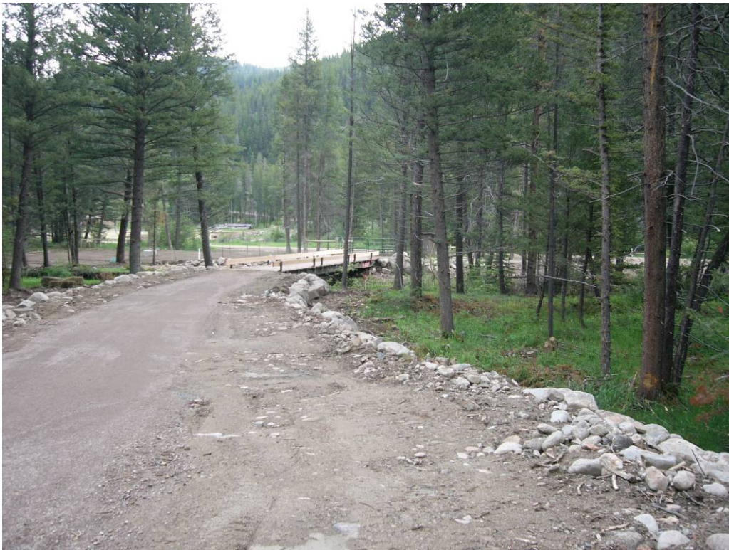
From road centerline of culvert crossing looking toward bridge and main channel.
