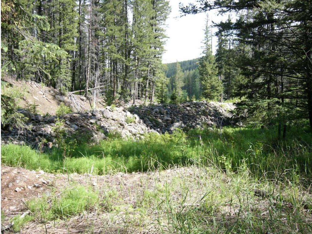
On right bank, same location as previous looking further downstream at main dike with 8 ft height compared to lower dike of 4 ft in upstream area.
