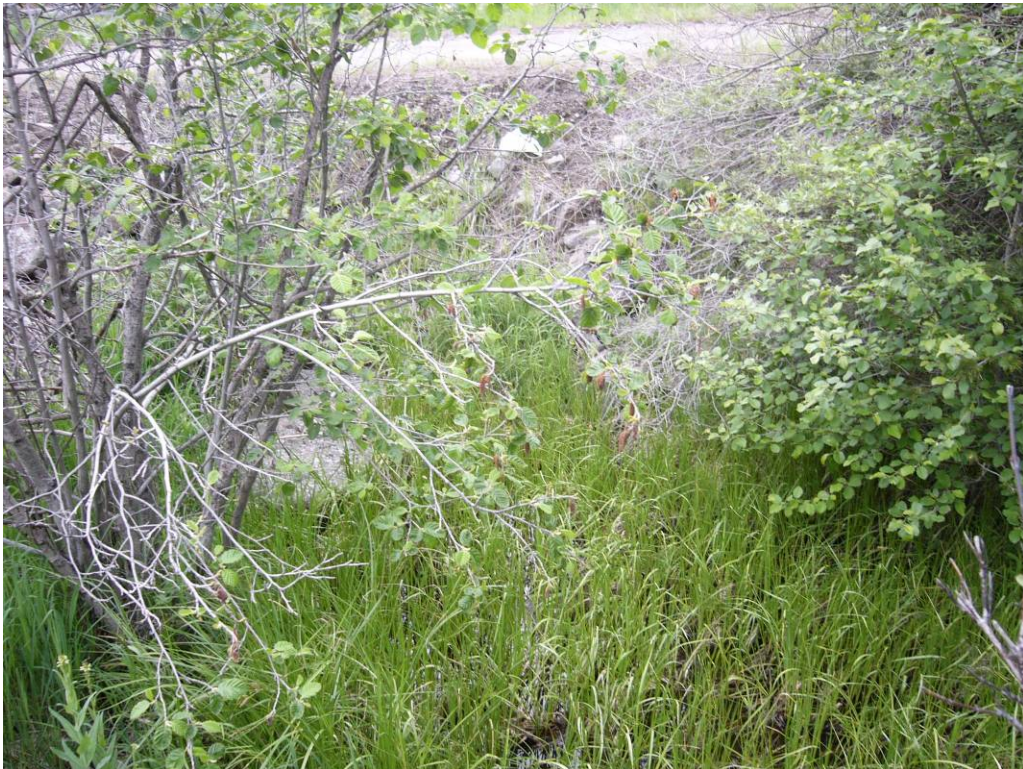
From channel looking at culvert entrance. Appeared to be an 12 to 18" culvert mostly blocked by vegetation and sediment. Culvert at base of slope near photo center. Top of road visible at photo top.
