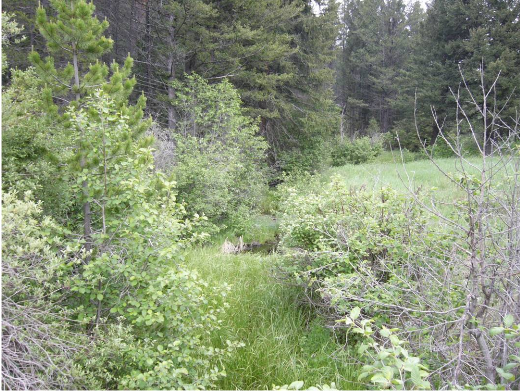
From Chessman road looking upstream at old channel above culvert entrance.
