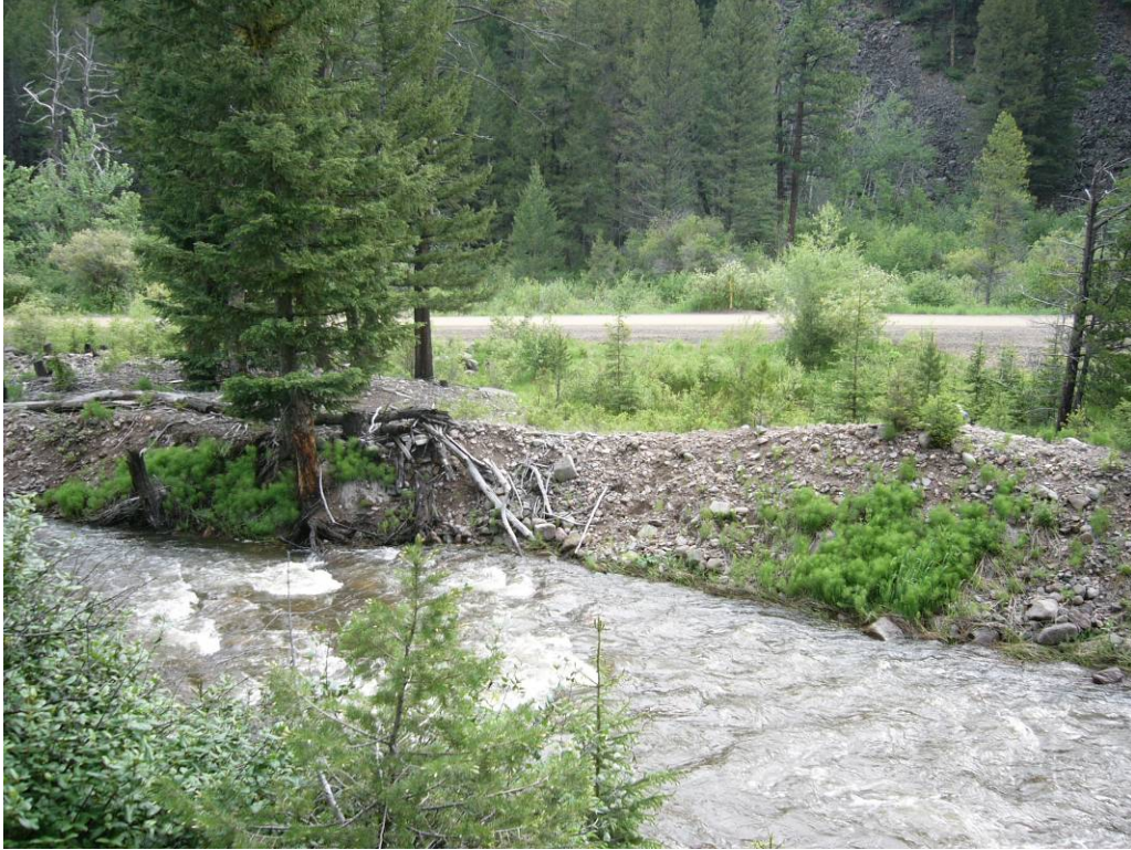
From top of left bank near XS#6, looking downstream with focus upstream of previous photo, looking at opposite bank and low saddle in rock berm. Evergreen tree area is natural high spot, near possible culvert location beneath Rimini Road for wetlands on east side.
