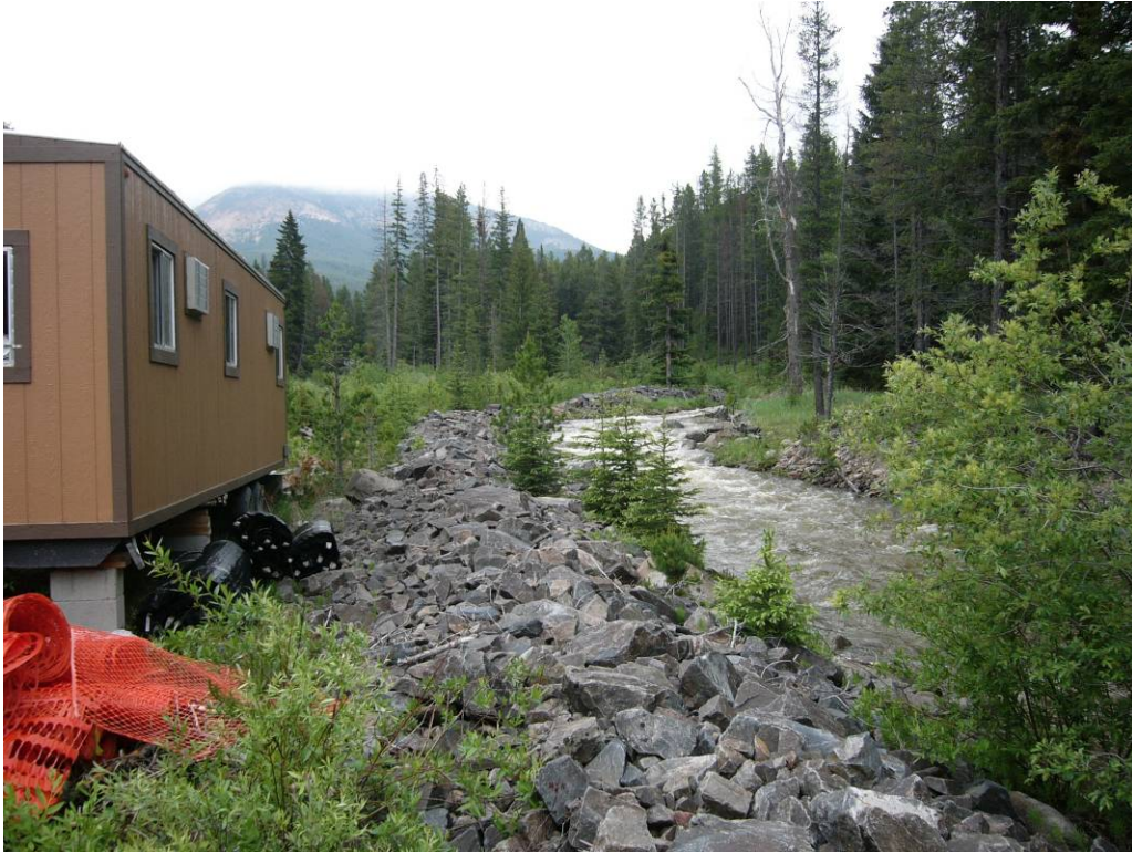
From right bank looking upstream at rock berm and work trailer.
