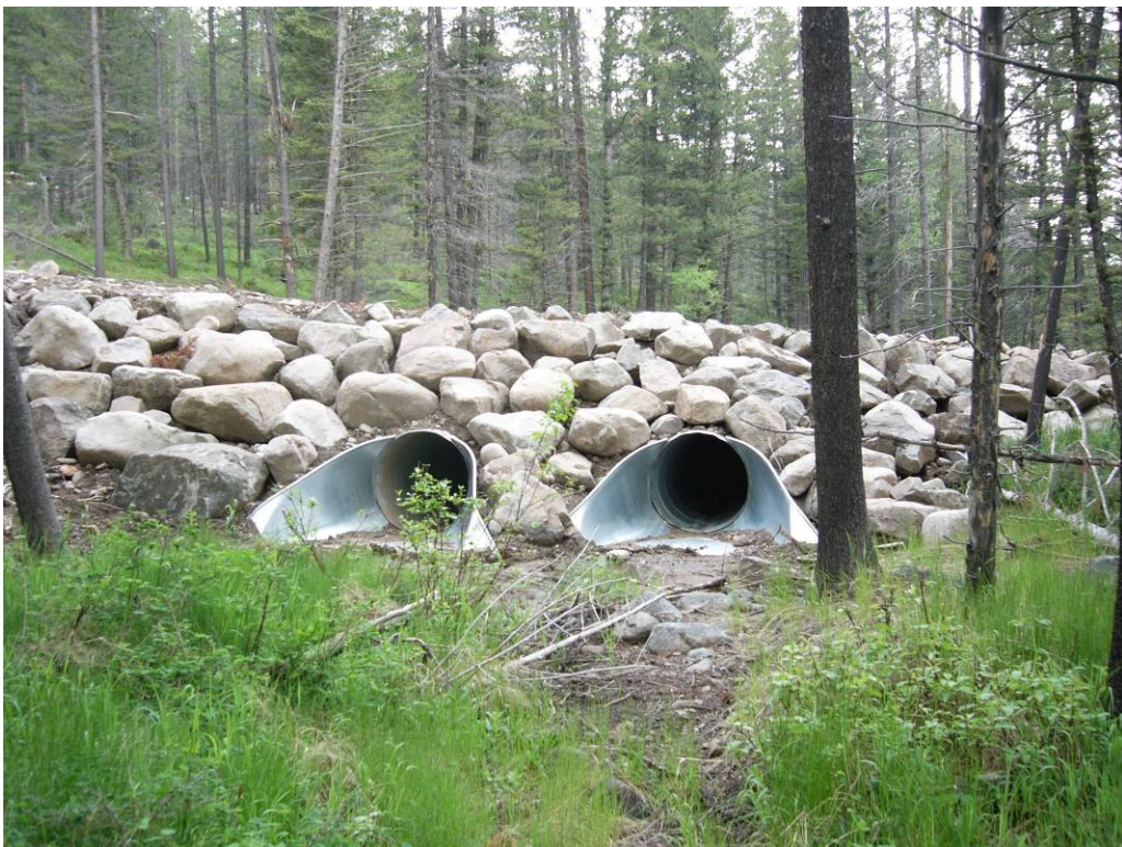
Two 42" diameter CMP beneath new road crossing that provides outlet for left bank overland flow.
