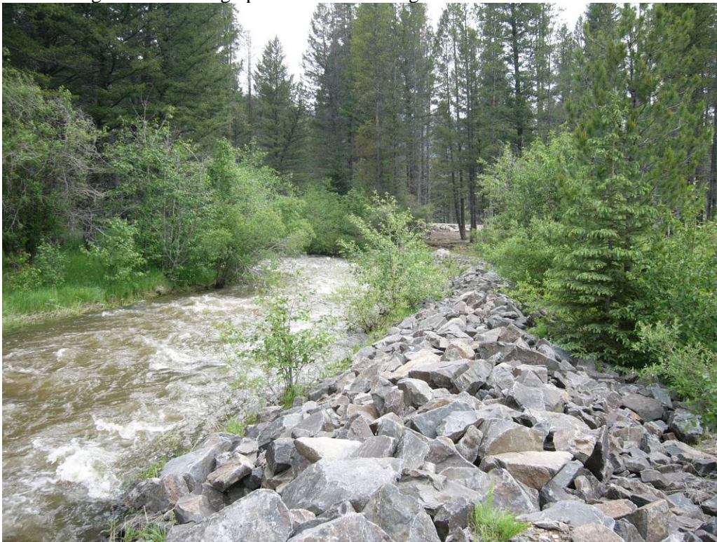
From right bank looking downstream at rock berm, just below trailer.
