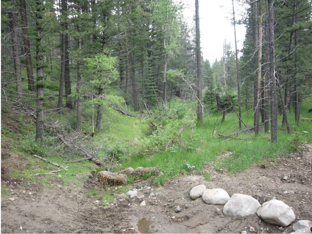
From road looking downstream at outlet for 2 42" culverts.
