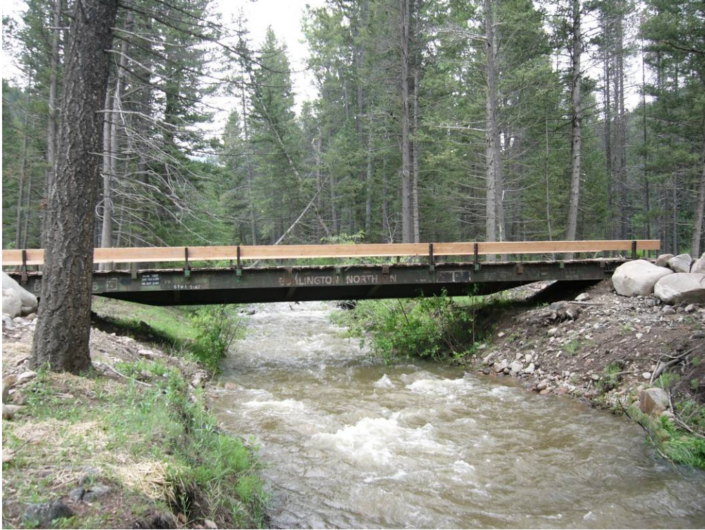
From downstream right bank looking upstream at new bridge.
