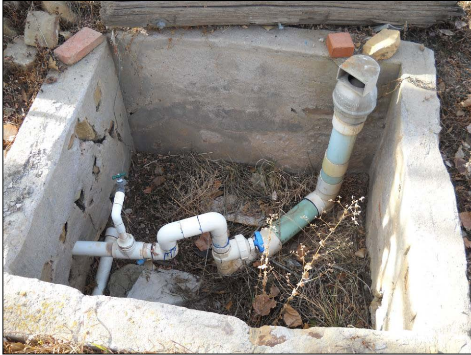
Figure 4.26. Air vent and water hookup near residence.
