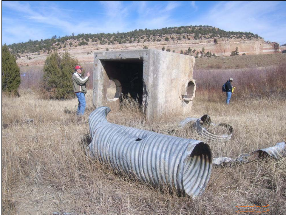
Figure 4.10. Large concrete diversion box removed from system, facing north. Note corrugated metal pipe fragments in foreground.
