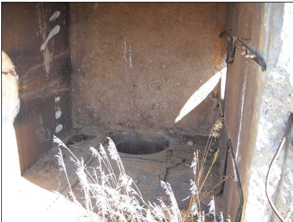
Figure 4.11. Interior of diversion box, facing northeast, showing rails for gate mechanisms and gouges from backhoe.
