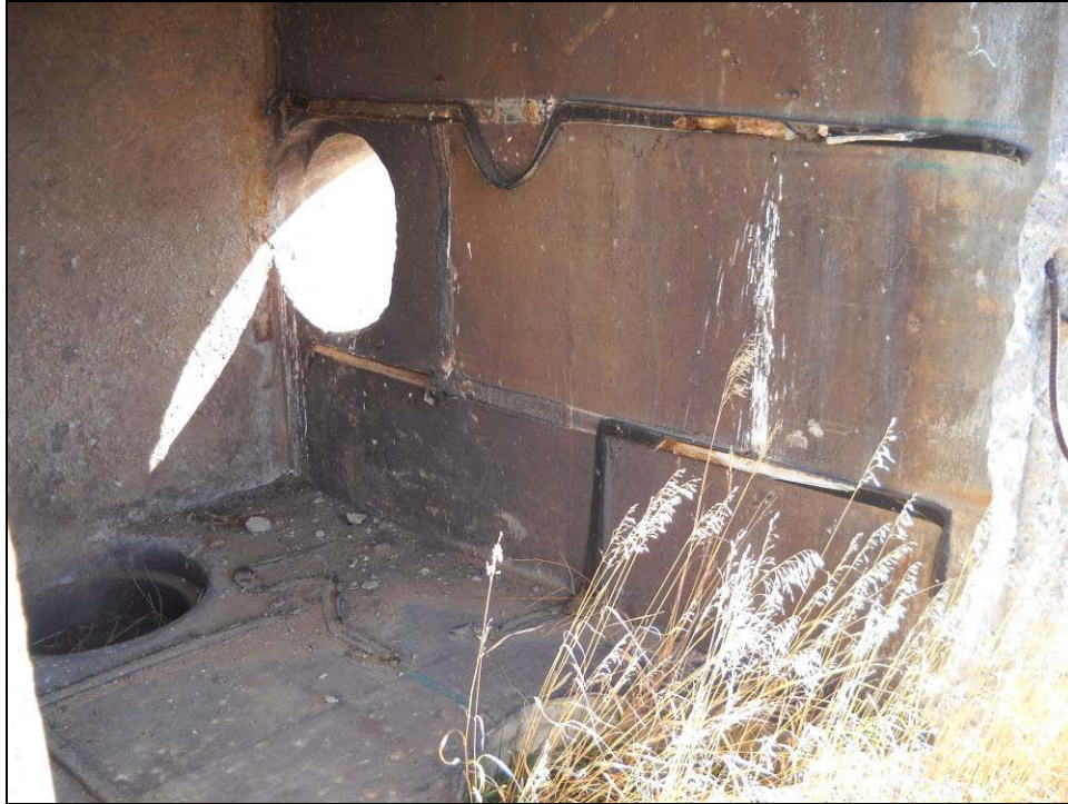
Figure 4.12. Interior of diversion box, facing east, showing rails for gate mechanisms.
