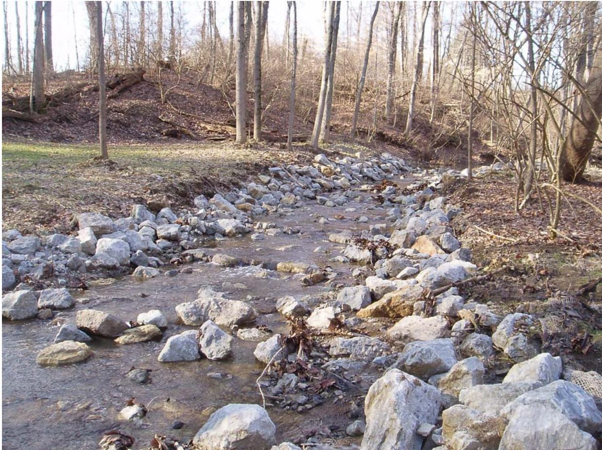
Figure 22 Sorting of trapezoidal riprap channels into rock clasts (Source: Alan Schlindwein).
