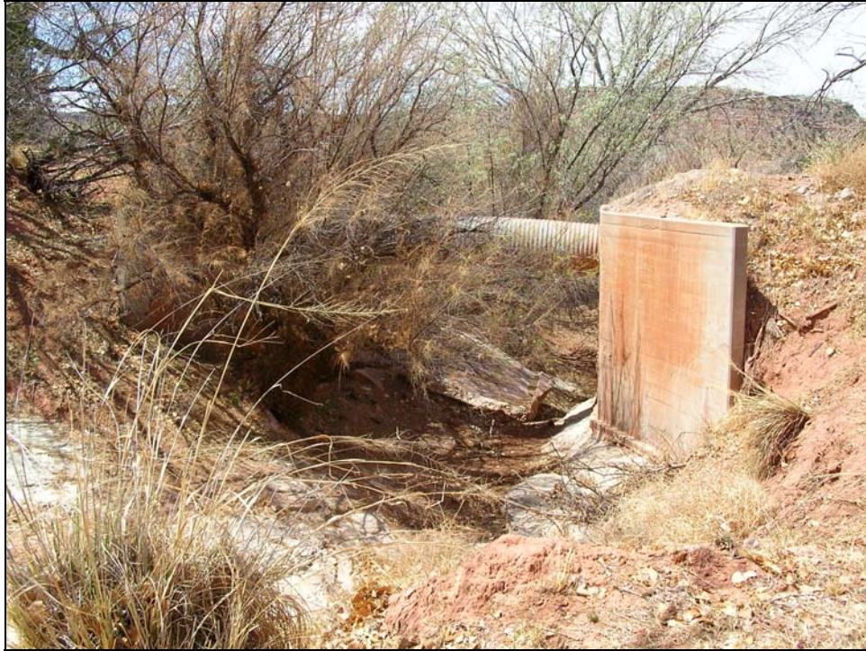
Figure 4.1. Overview Photograph of Flume No. 1 to be by-passed and abandoned in place. Photograph No. 9889.
