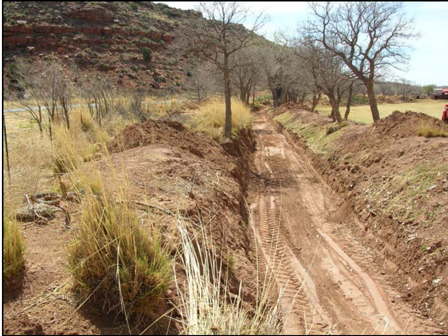
Photograph No. 9785: Overview of existing ditch alignment with example of upland sediment removed from ditch. East Puerto de Luna Acequia Irrigation Pipeline Project, approximately 7-miles southeast of Santa Rosa, Guadalupe County, New Mexico. Photograph by Corps' Archaeologist Gregory D. Everhart, April 14, 2009.
