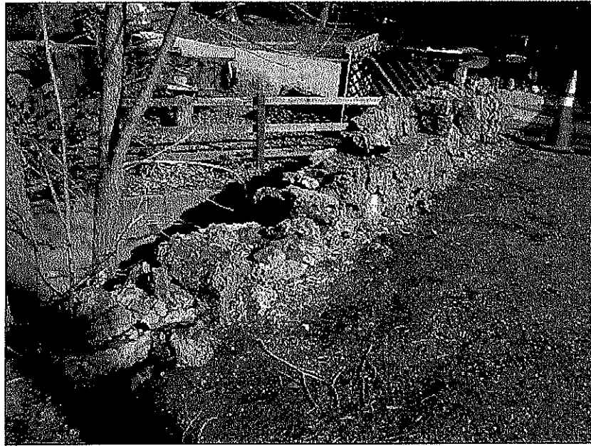
Typical condition of railing with missing stones, deteriorated and missing mortar
