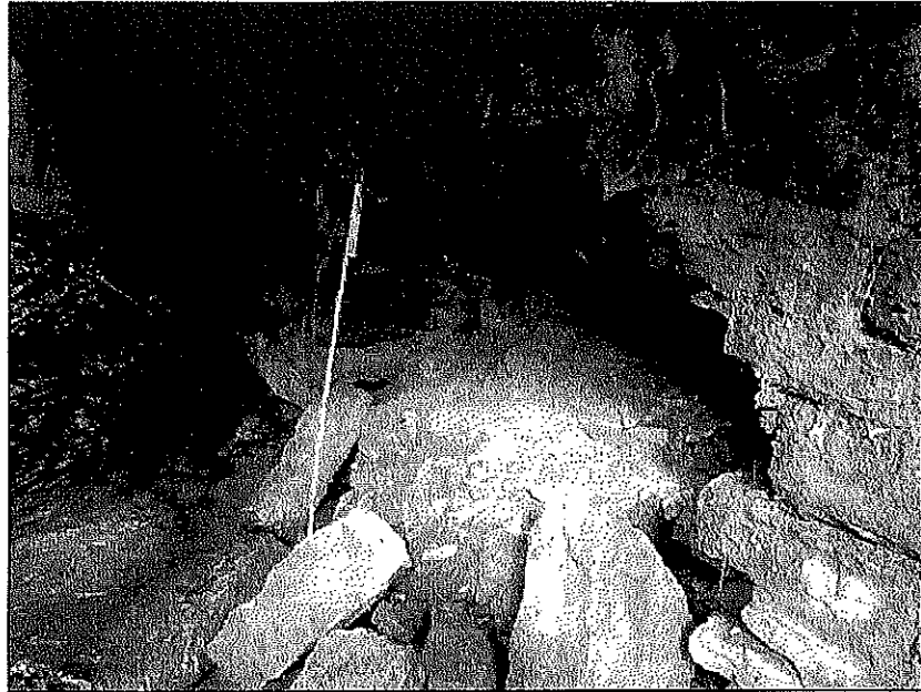
7'-0" long x 4'-0" high x 3'-0" deep (horizontal penetration) collapsed section of arch barrel at the north (close-up)
