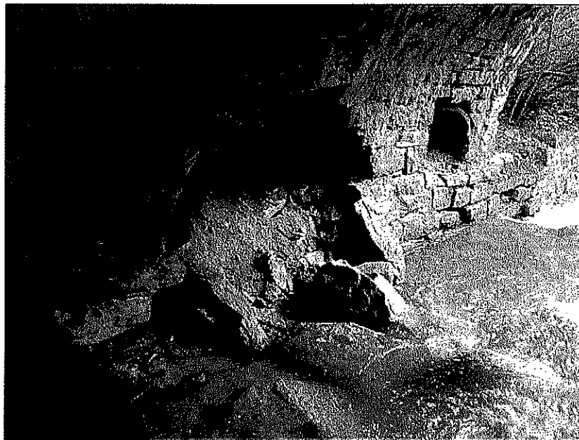
7'-0" long x 4'-0" high x 3'-0" deep (horizontal penetration) collapsed section of arch barrel at the north
