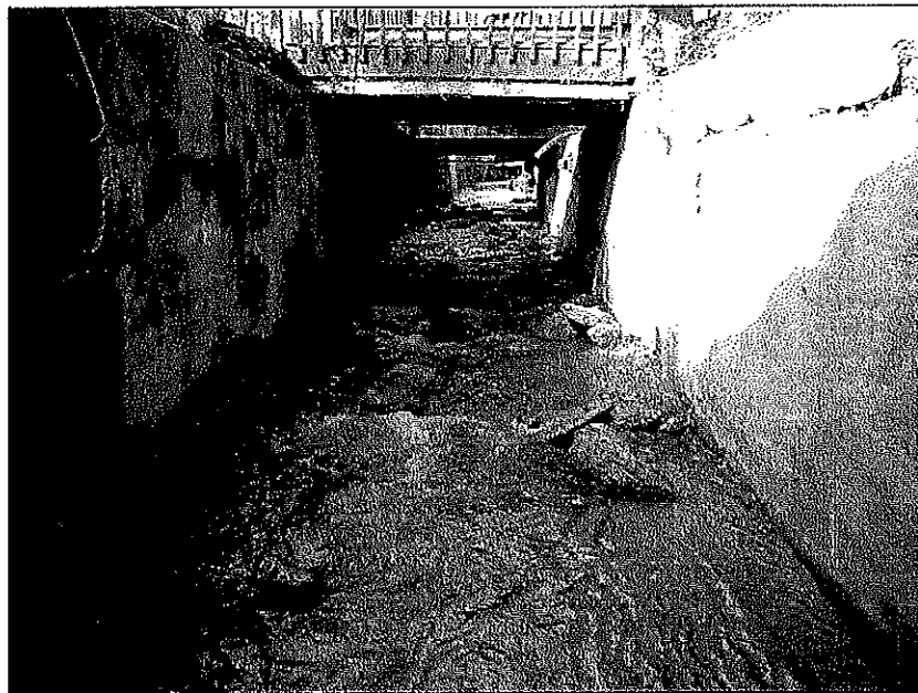
Channel looking upstream; note the exposed footing along the south retaining wall
