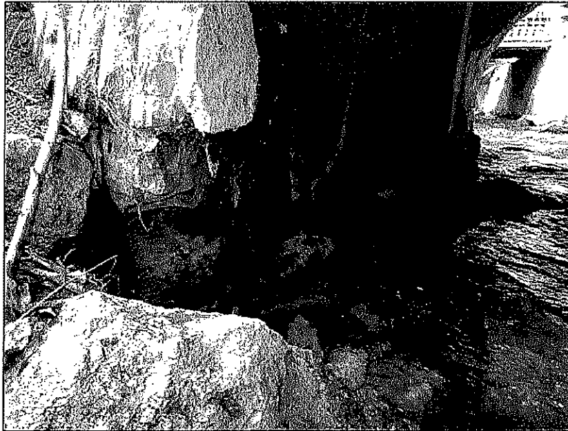
12'-0" long x 3'-0" high x 2'-0" deep (horizontal penetration) collapsed section of arch barrel at the south (close-up view)
