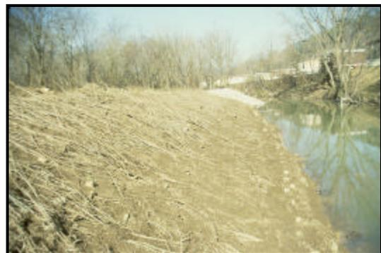
**Figure 7. Brush mattress after light backfill of soil**
