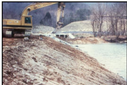
**Figure 3. Slope the bank to provide an even surface for the brush mattress**
