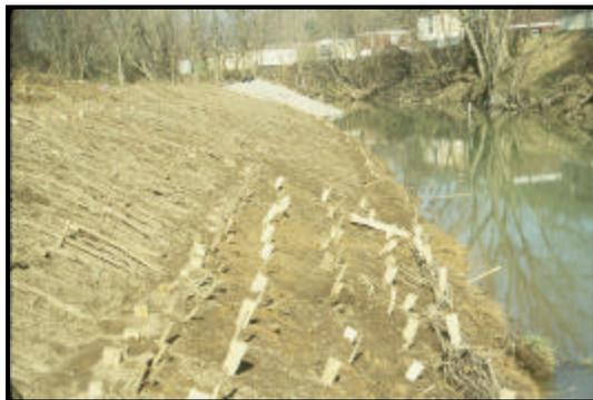
**Figure 4. Double row of brush mattress showing stake placement**
