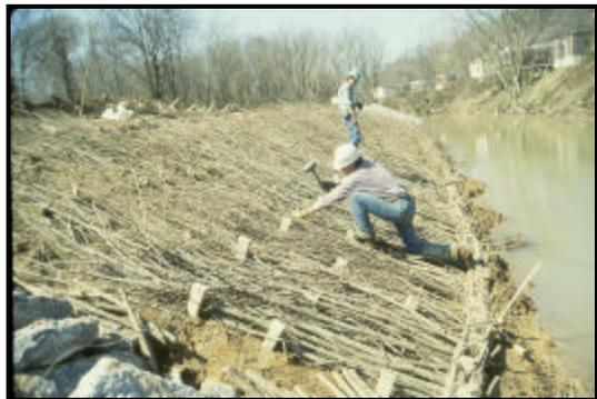
**Figure 6. Securing a brush mattress with stakes and twine**
