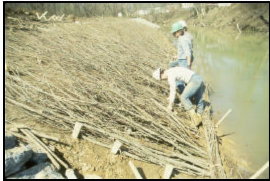
**Figure 5. Branch placement beneath live fascine and against bank face**
